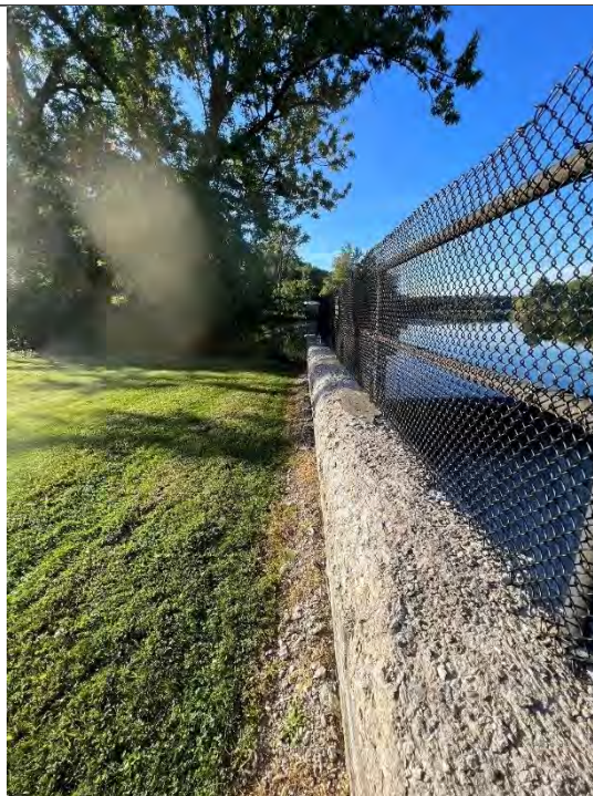
Photo No. 72 – Concrete Deterioration Top of Downstream Right Wall Upstream of M-52 Bridge Looking Upstream
