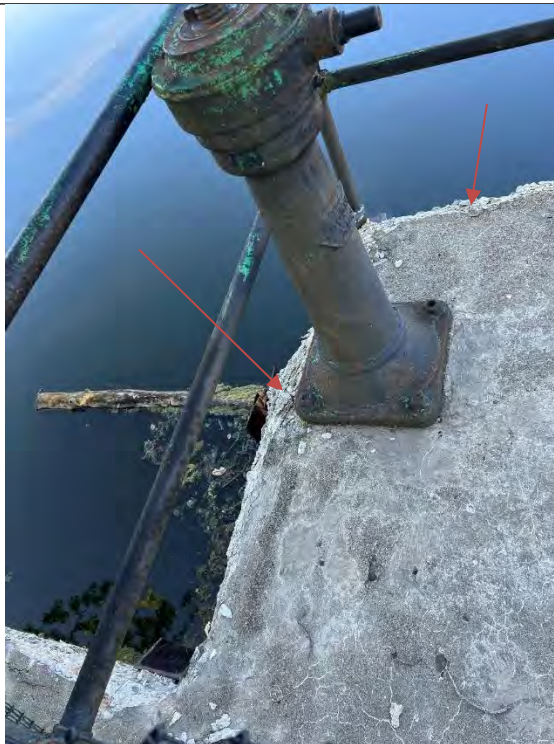
Photo No. 22 – Concrete Deterioration on Left and Upstream Side of Right Operator Deck
