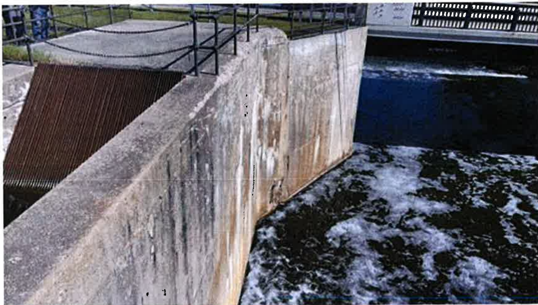
Photo #46 - Left downstream spillway abutment wall. Efflorescence present. Spalling present at the top of the wall. Cracking and loss of concrete observed near the bottom of the wall
