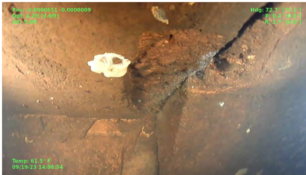
Figure 24 – Upstream, Intake Tunnels East Wall: Spalling on Ceiling
