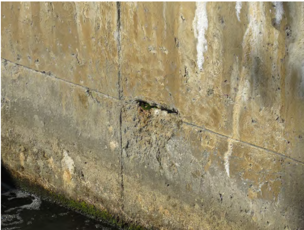
Figure 9 – Downstream, West Wall: Spalling
