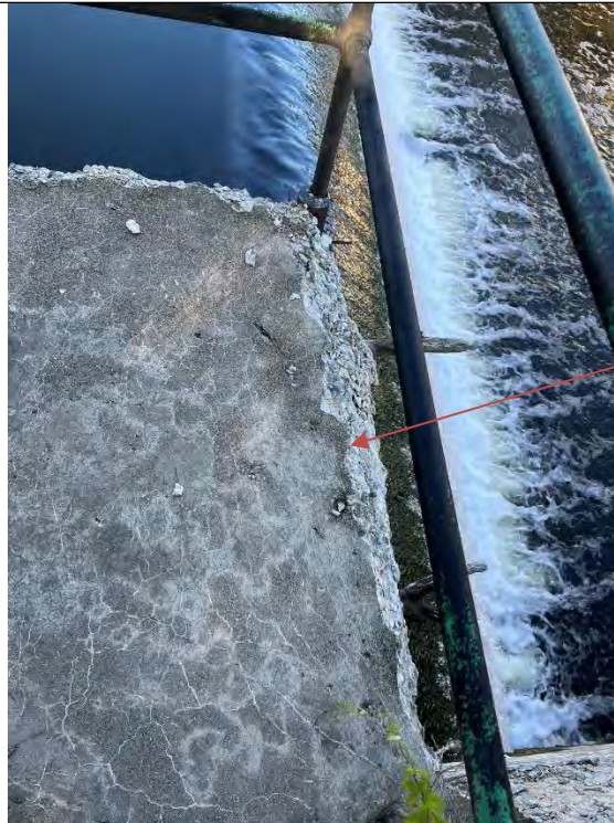
Photo No. 23 – Concrete Deterioration on Downstream Side of Right Operator Deck
