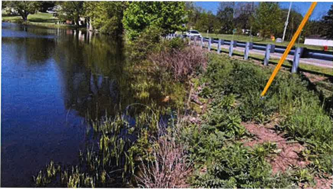
Photo #3 - Upstream slope of left embankment. Brush and trees present
