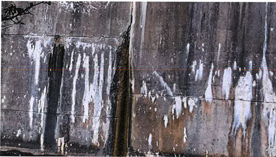
Photo #80 - Seepage areas on left downstream wall
