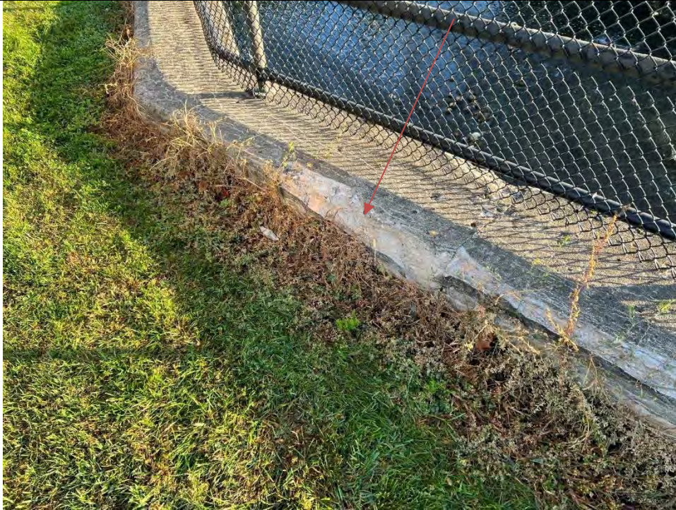
Photo No. 57 – Concrete Deterioration at Top of Downstream Left Wall Downstream of M-52 Bridge Looking Downstream
