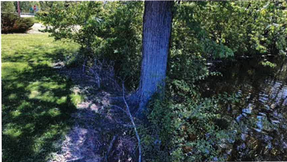
Photo #9 - Upstream slope of right embankment. Tree and brush present towards end of embankment
