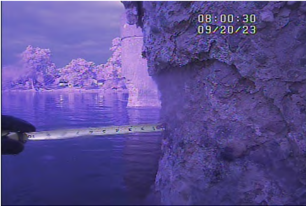
Figure 34 – Upstream, Intake Tunnel, Bullnose 1: Concrete Loss
