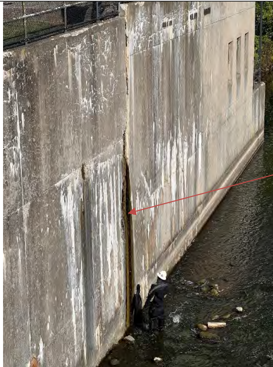
Photo No. 49 – Concrete Deterioration and Leaking at Construction Joint on Downstream Left Wall Downstream of M-52 Bridge
