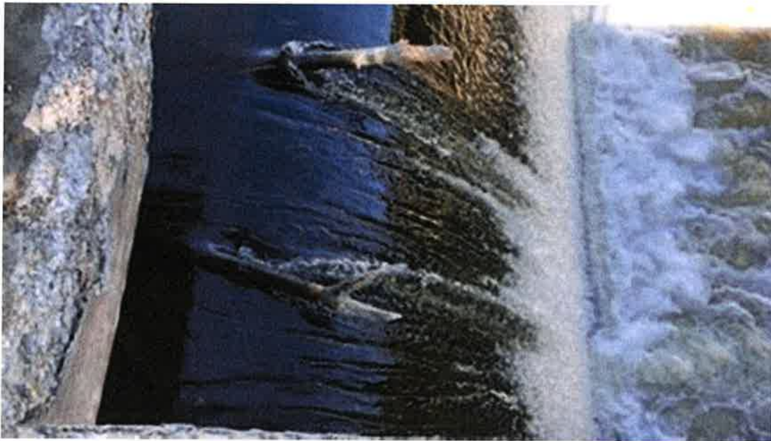
Photo #71 - Spillway crest at right drawdown gate. Drawdown outlet was unable to be observed
