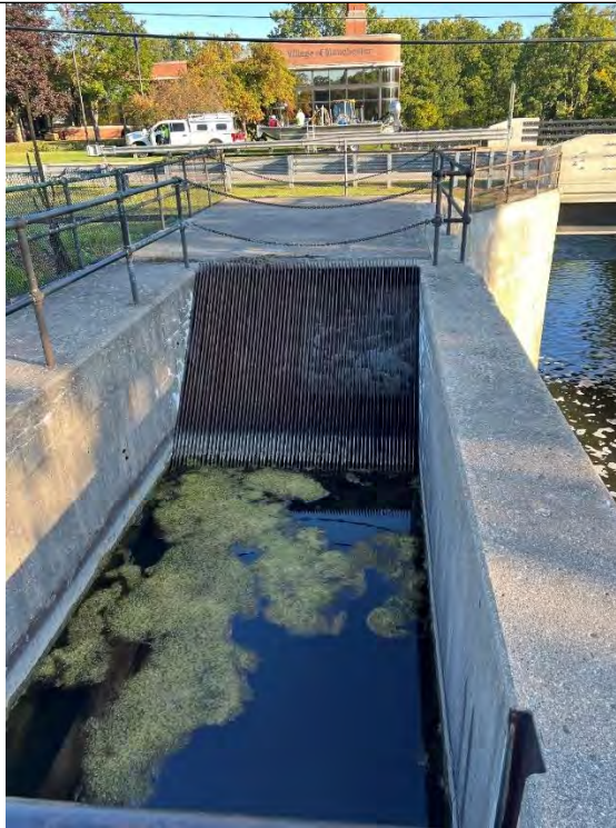
Photo No. 37 – Trashrack Upstream of Penstock Looking Downstream
