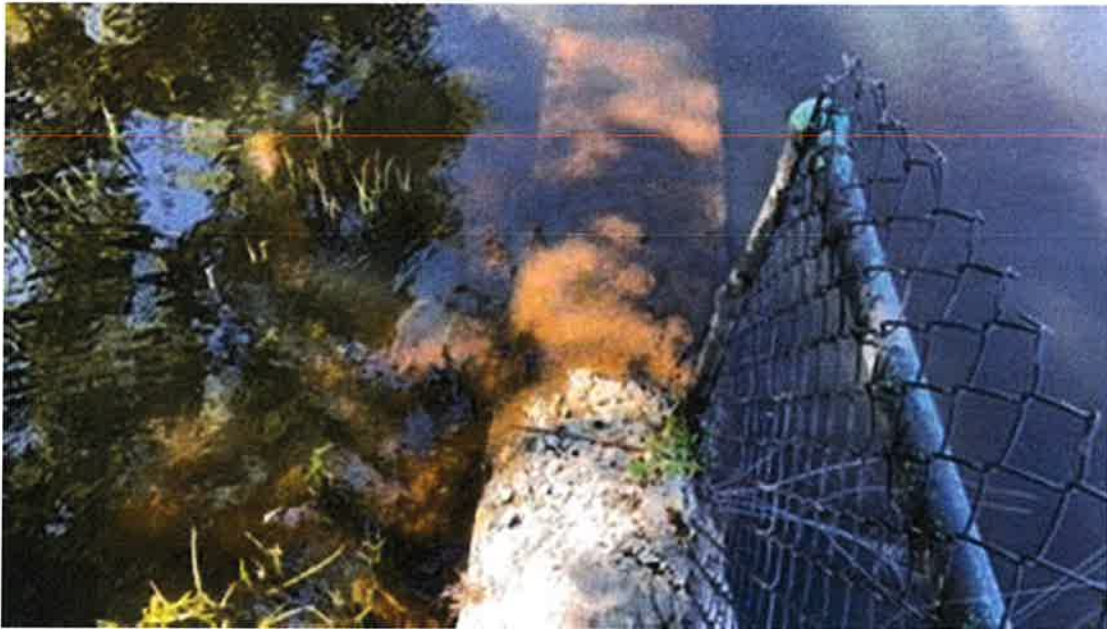
Photo #64 - Top of spillway's right upstream abutment wall. Loss of concrete at waterline
