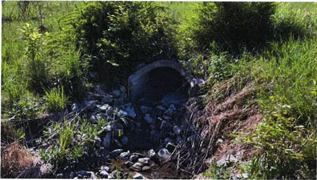
Photo #31 - Storm sewer outfall on right embankment downstream slope
