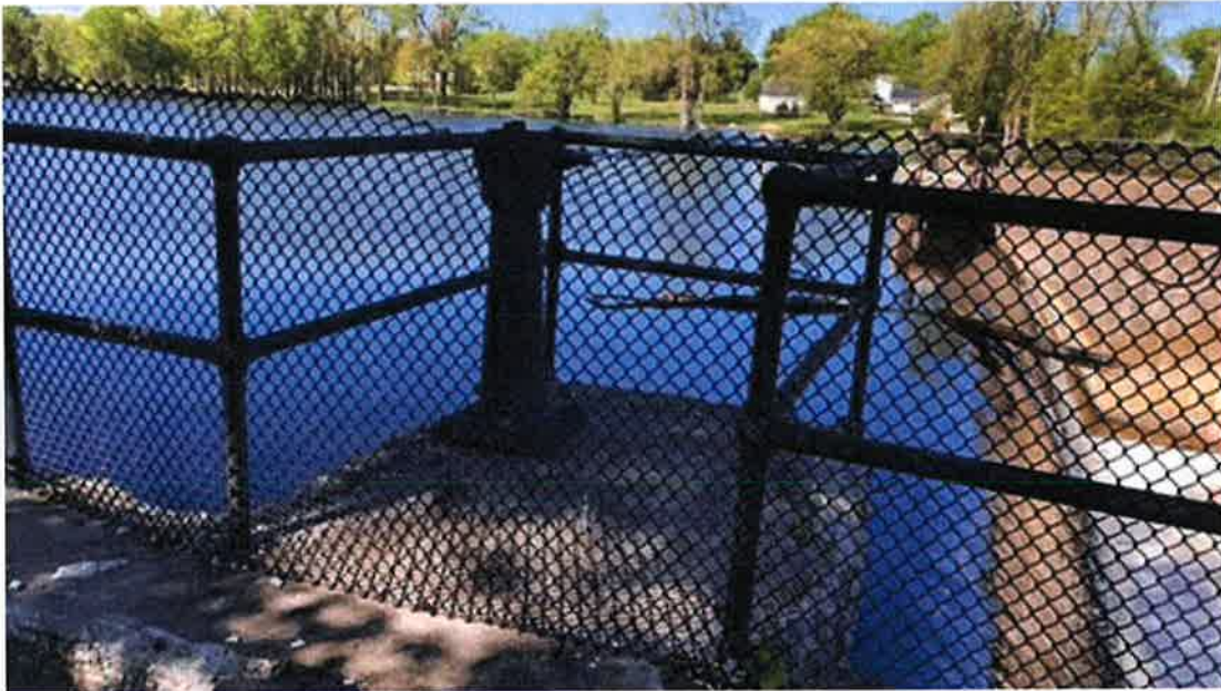
Photo #69 - Right drawdown gate operator
