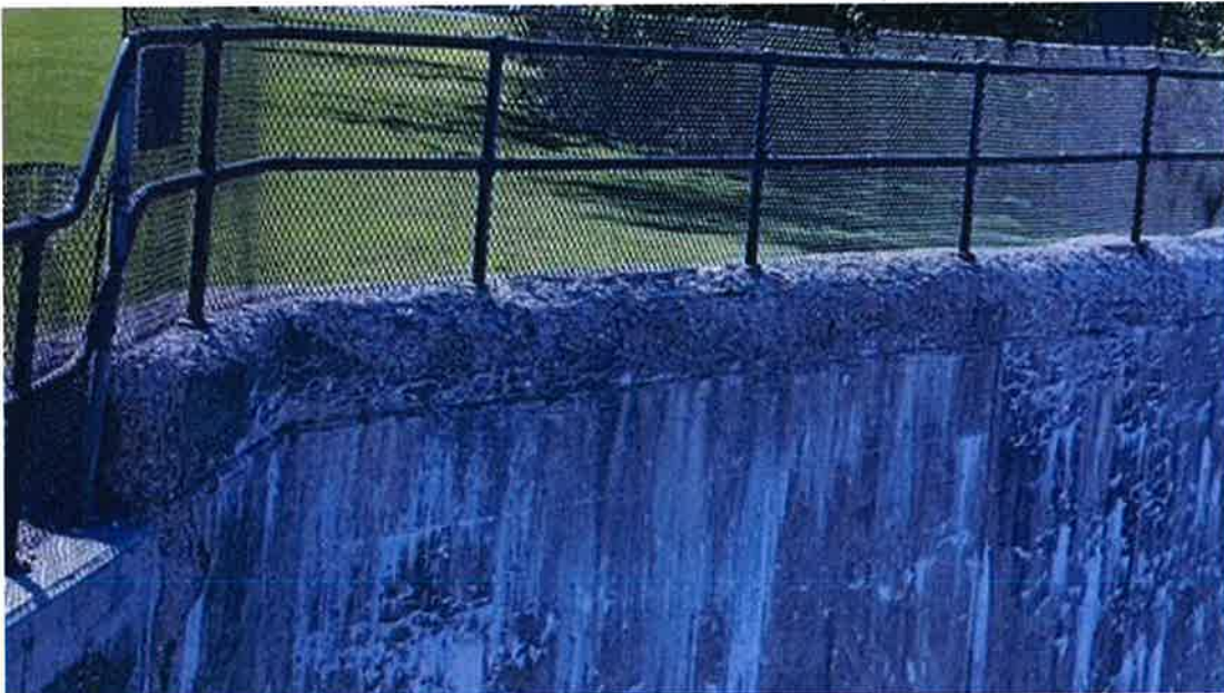
Photo #58 - Spalling on top of the spillway's right downstream abutment wall
