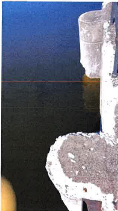
Photo #92 - Powerhouse sluiceway inlet. Concrete shows severe spalling at piers
