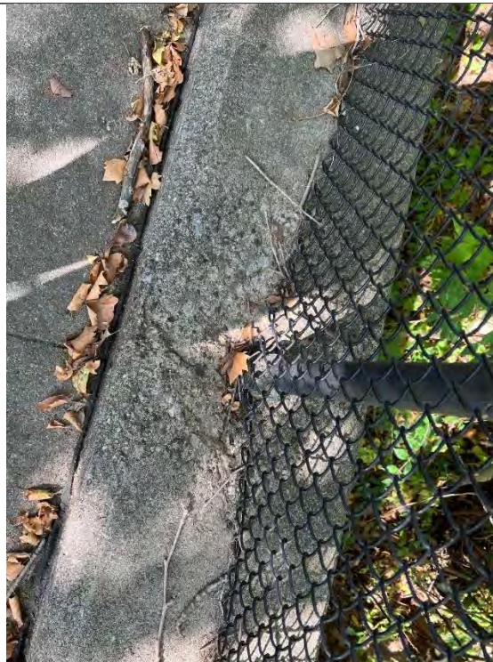
Photo No. 90 – Concrete Deterioration at Top of Seating Area Wall Looking Left
