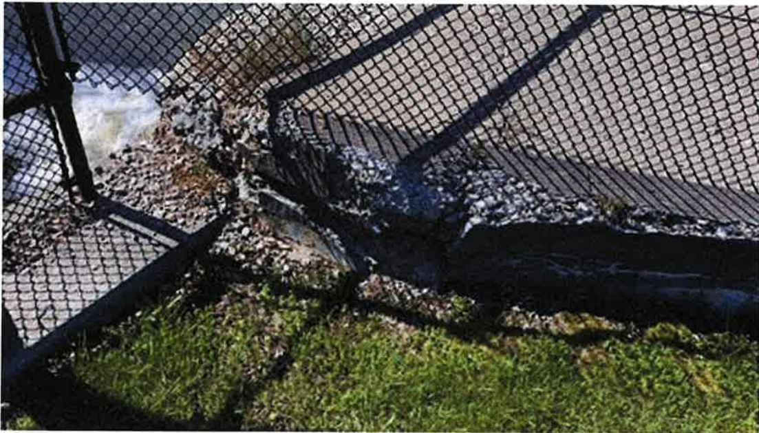
Photo #51 - Concrete deterioration at spillway deck over sluiceway
