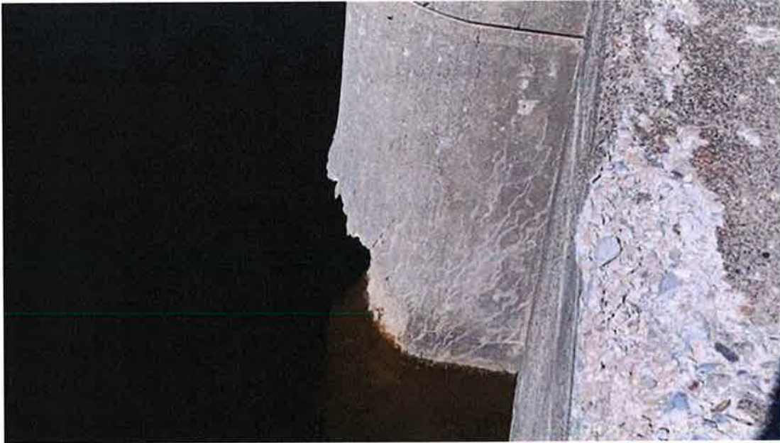
Photo #93 - Loss of concrete at waterline of powerhouse sluiceway inlet, left side
