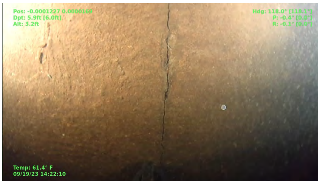
Figure 27 –Upstream, Intake Tunnels East Wall: Hairline Crack
