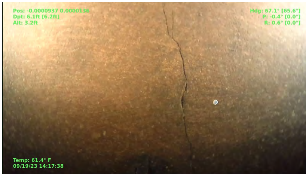
Figure 26 –Upstream, Intake Tunnels East Wall: Hairline Crack
