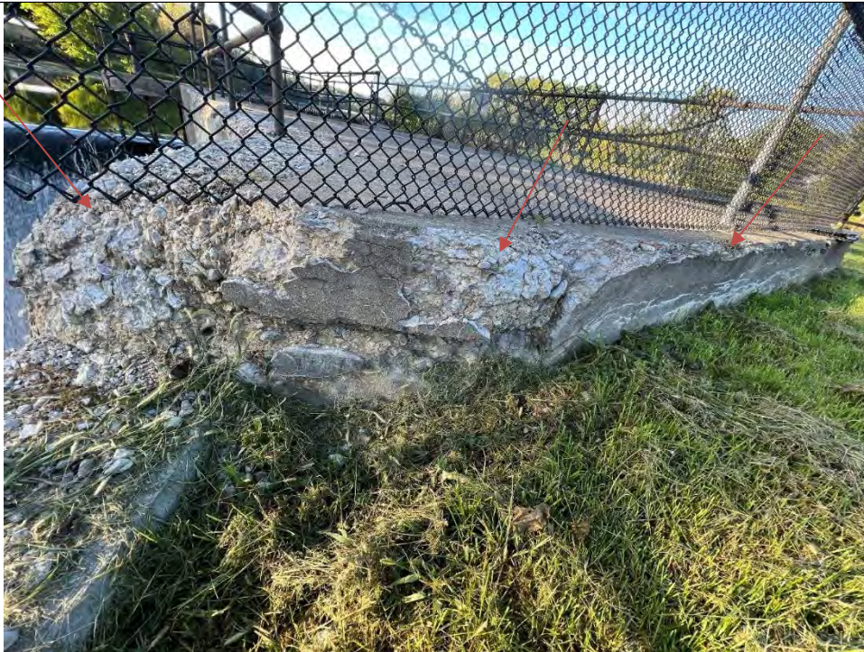
Photo No. 28 – Concrete Deterioration on Downstream Side of Penstock Intake Deck Looking Upstream
