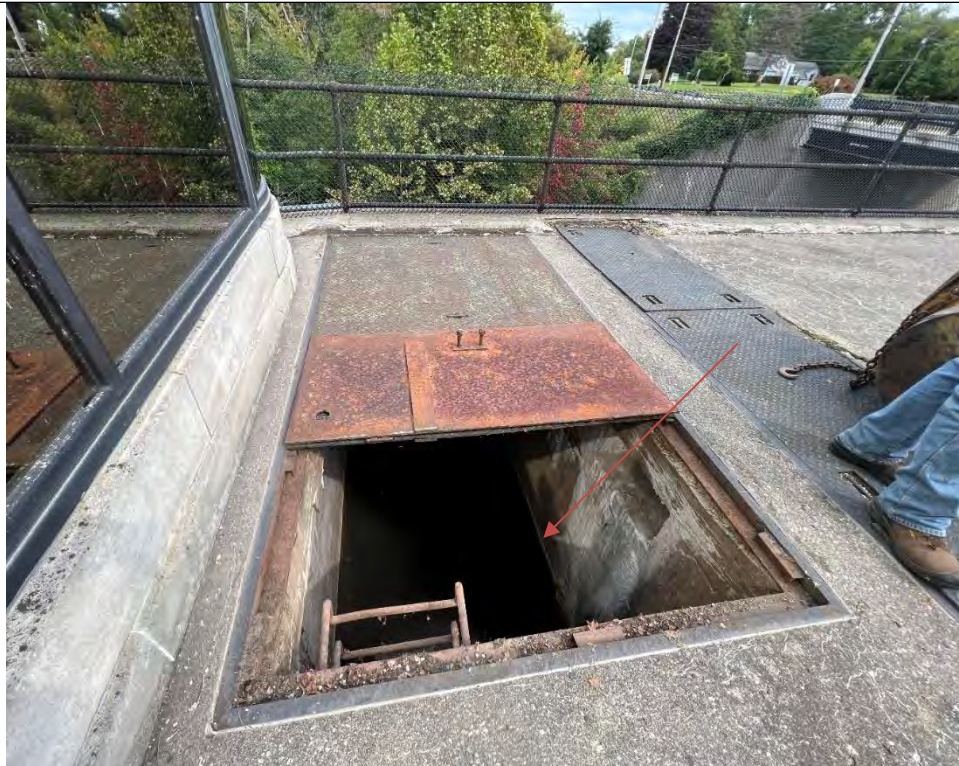
Photo No. 79 – Access to Turbine Vaults Upstream of Powerhouse
