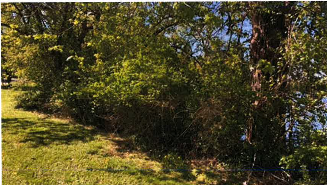
Photo #10 - Upstream slope of right embankment. Tree and brush present towards end of embankment
