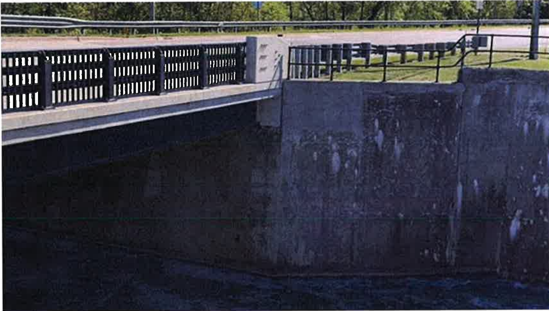
Photo #57 - Right downstream spillway abutment wall at joint with bridge. Efflorescence present throughout, spalling present at the top of the wall
