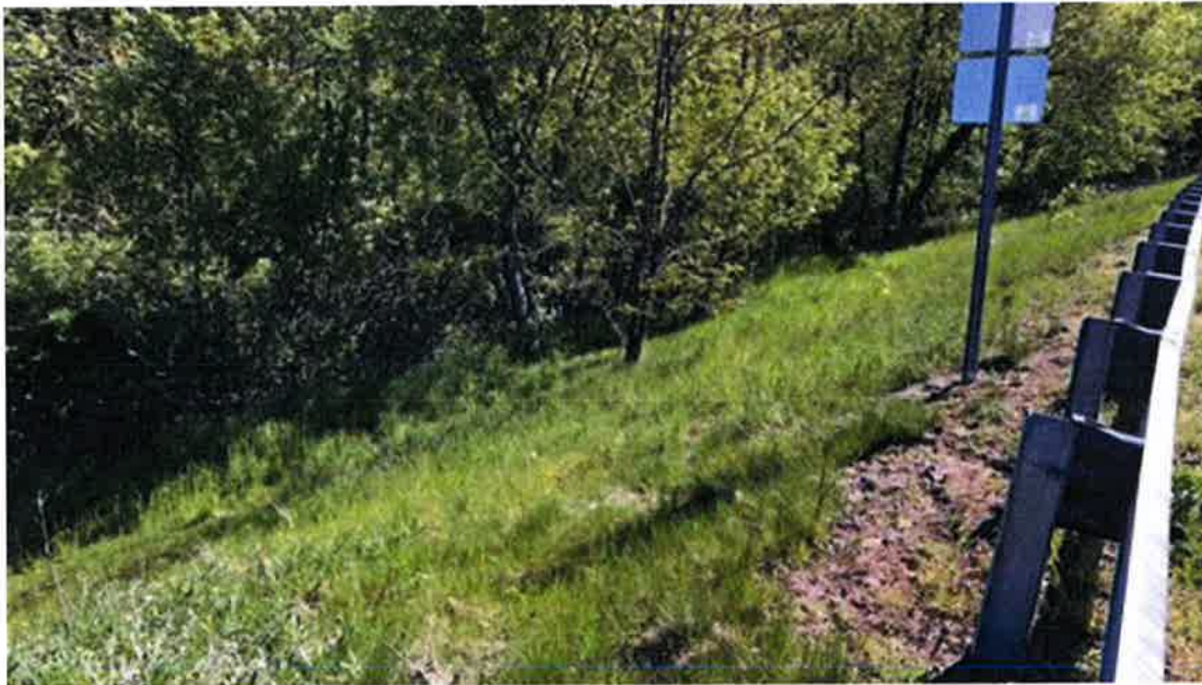
Photo #26 - Downstream slope of right embankment viewed from crest. Trees and brush encroaching past groin and past toe
