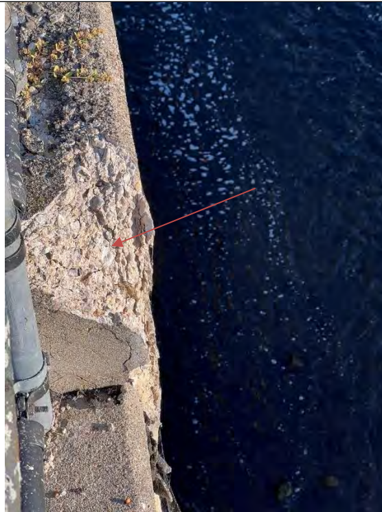
Photo No. 63 – Concrete Deterioration on Top of Downstream Left Wall Upstream of Powerhouse Looking Downstream
