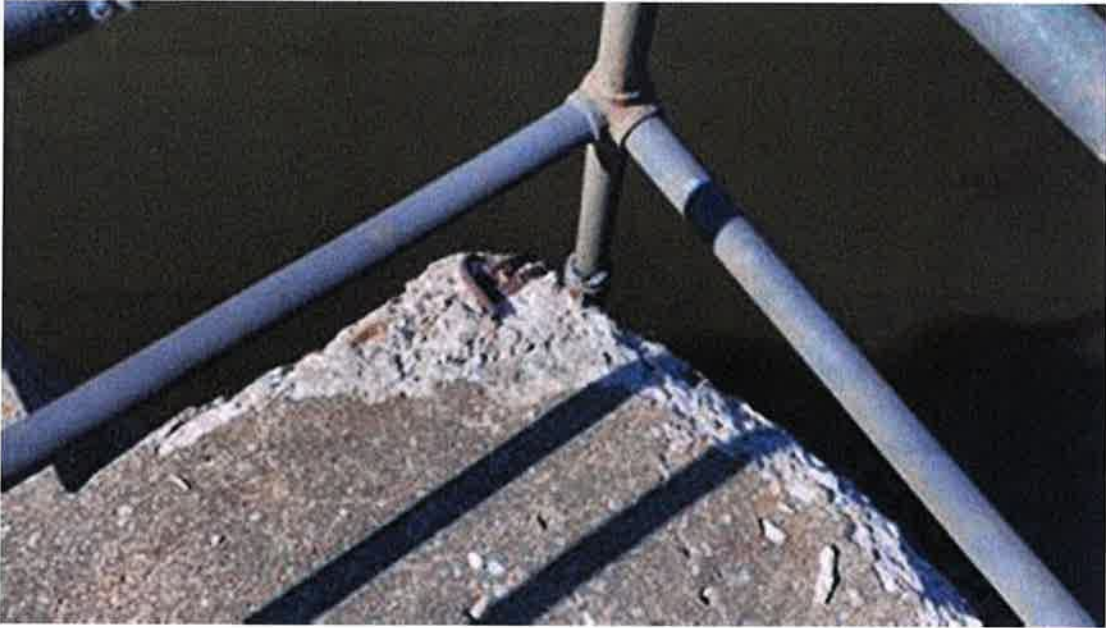
Photo #67 - Spalling, exposed rebar at left spillway gate operator deck. Guardrail connection to concrete is compromised
