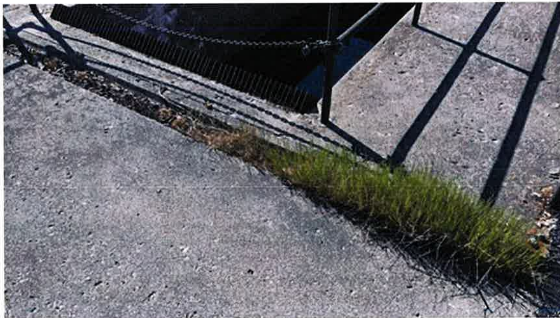
Photo #50 - Some vegetation growing within concrete spillway structure that should be removed
