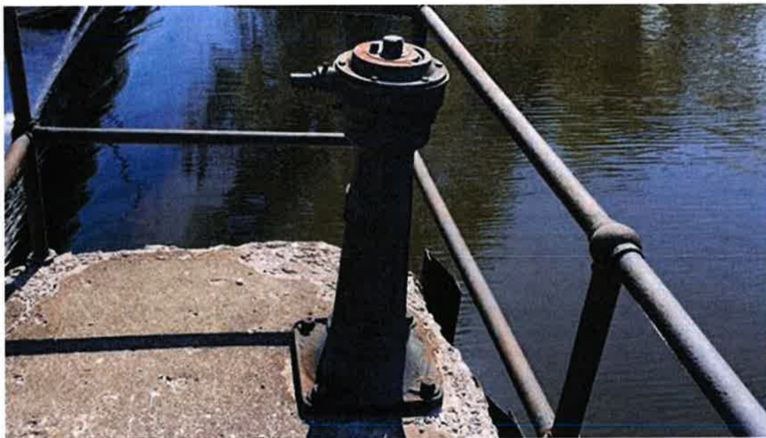
Photo #66 - Left drawdown gate operator. Note severe deterioration of concrete on operator deck
