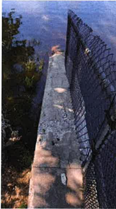
Photo #63 - Top of spillway's right upstream abutment wall. Minor spalling observed
