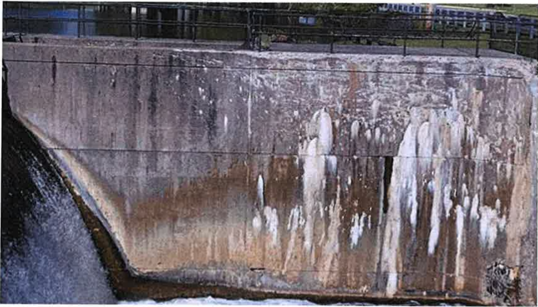
Photo #43 - Left downstream spillway abutment wall. Efflorescence present throughout. Some minor seepage observed at darker area of concrete
