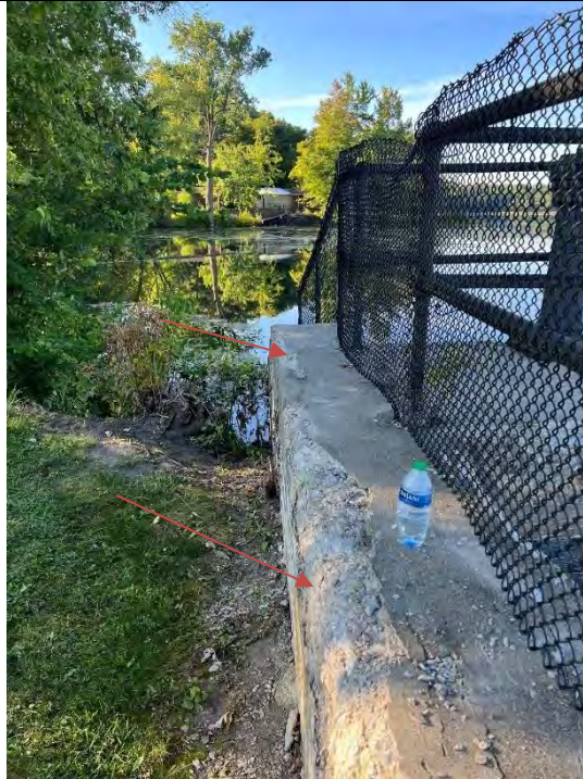
Photo No. 73 – Concrete Deterioration Top of Downstream Right Wall Upstream of M-52 Bridge Looking Upstream
