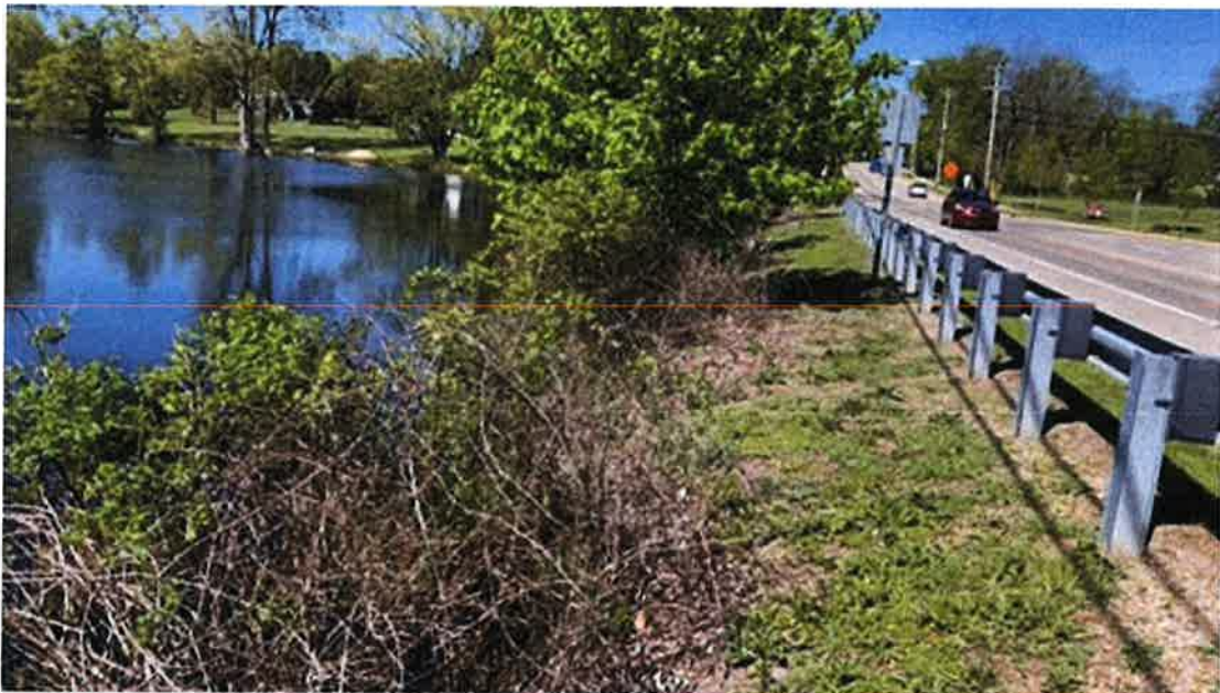
Photo #4 - Upstream slope of left embankment. Some trees and brush present on embankment near the waterline
