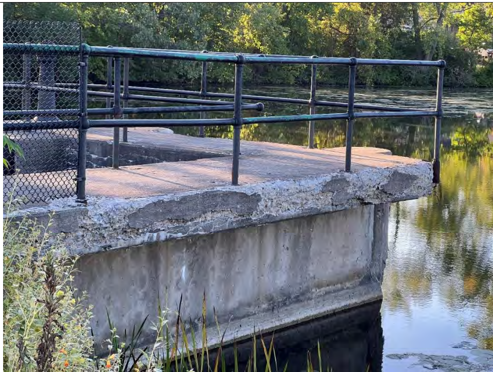
Photo No. 32 – Concrete Deterioration of Left Side of Penstock Intake Deck Looking Right
