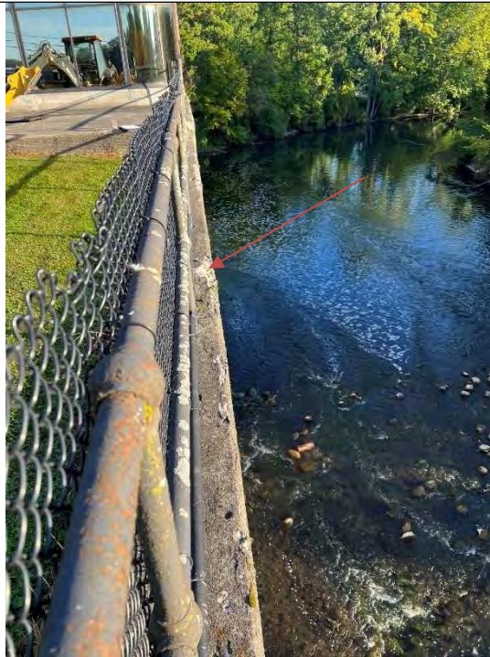
Photo No. 61 – Concrete Deterioration on Top of Downstream Left Wall Downstream of M-52 Bridge Looking Downstream
