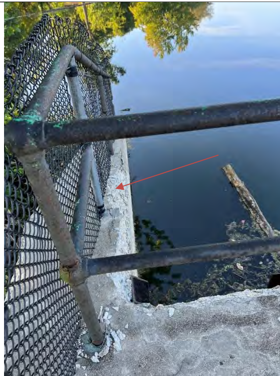
Photo No. 16 – Concrete Deterioration on Top of Upstream Right Wing Wall
