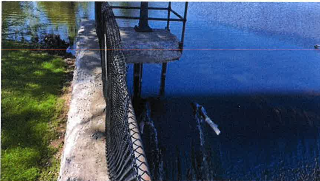
Photo #60 - Spalling on top of the spillway's right downstream abutment wall and gate operator deck
