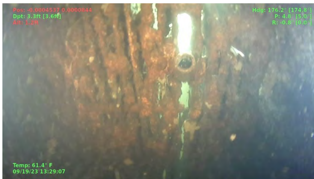
Figure 19 – Upstream, Intake Tunnels: Trash Rack
