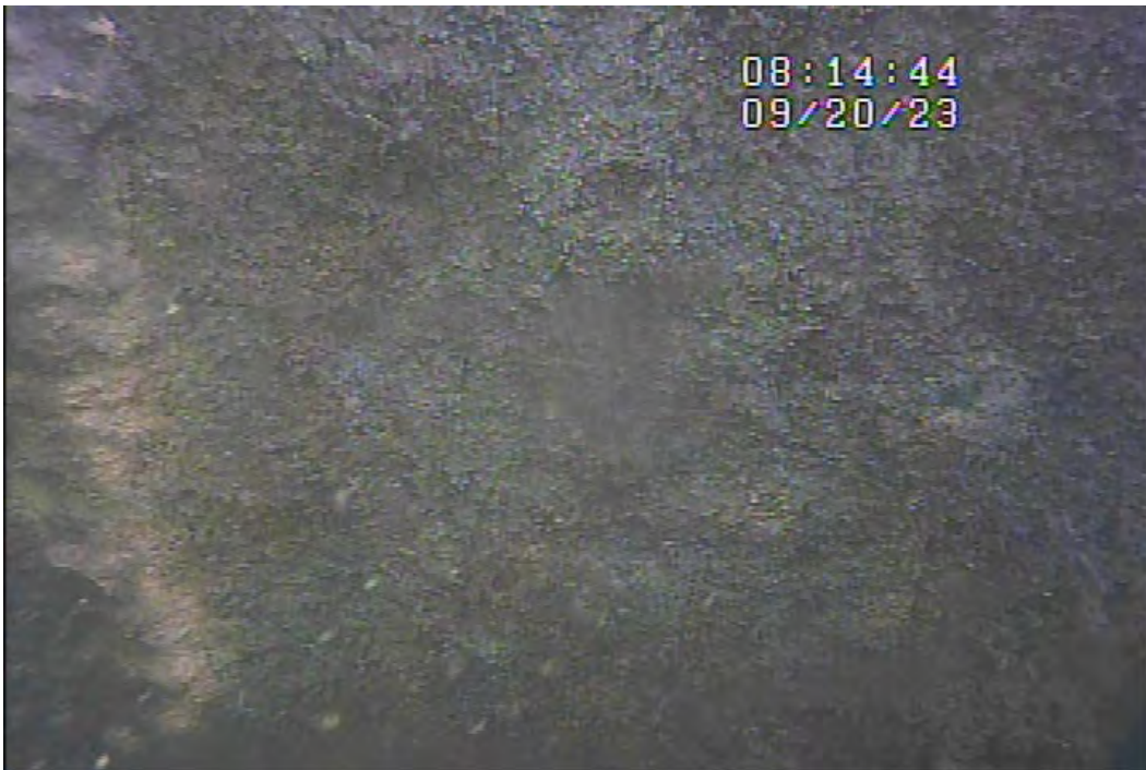
Figure 37 – Upstream, Intake Tunnel Bullnose 2: Scaling
