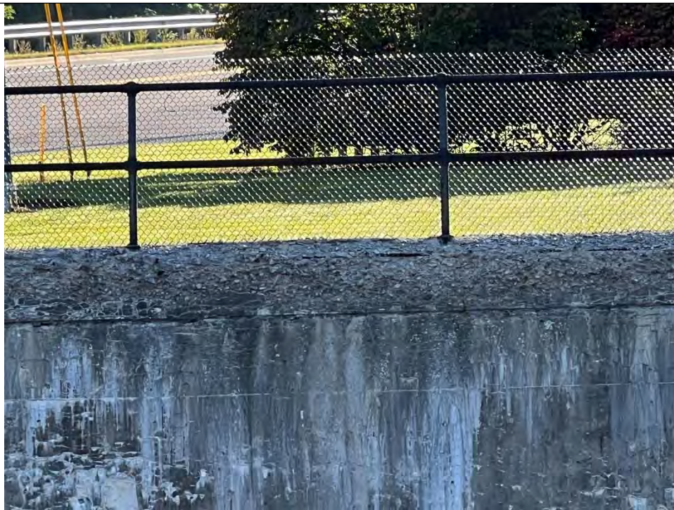
Photo No. 66 – Concrete Deterioration at Top of Downstream Right Wall Upstream of M-52 Bridge Looking Right
