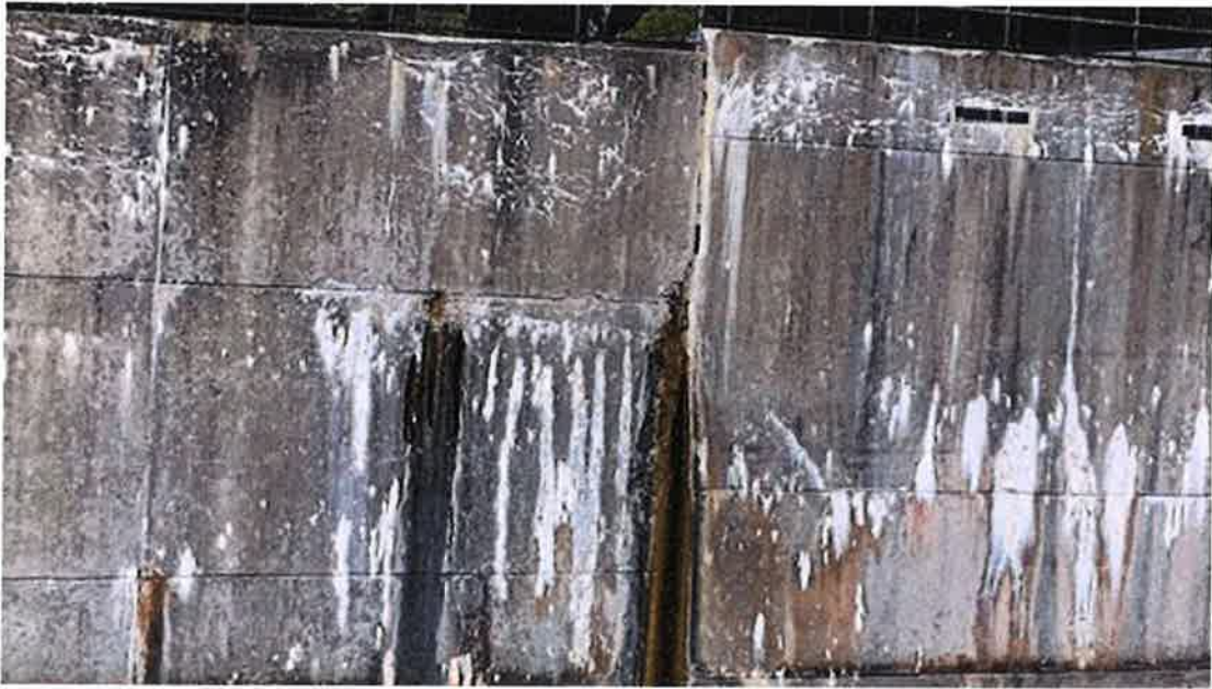
Photo #79 - Seepage in left downstream abutment wall
