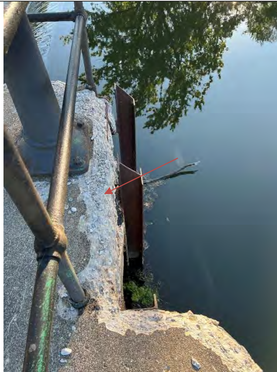
Photo No. 19 – Concrete Deterioration on Upstream Side of Left Operator Deck
