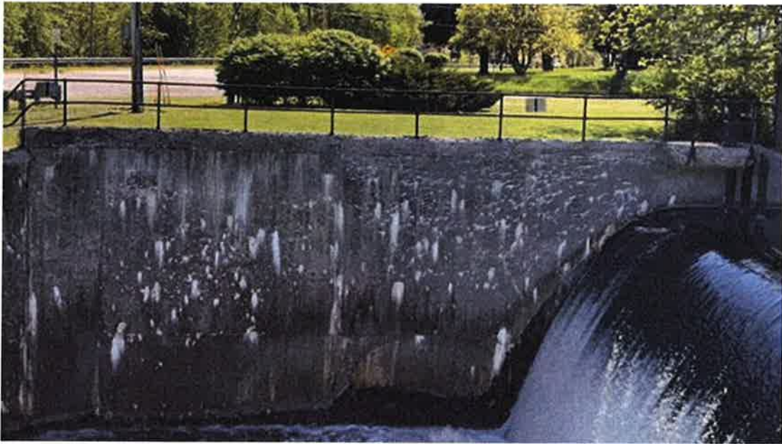
Photo #55 - Right downstream spillway abutment wall. Efflorescence present throughout, spalling present at the top of the wall
