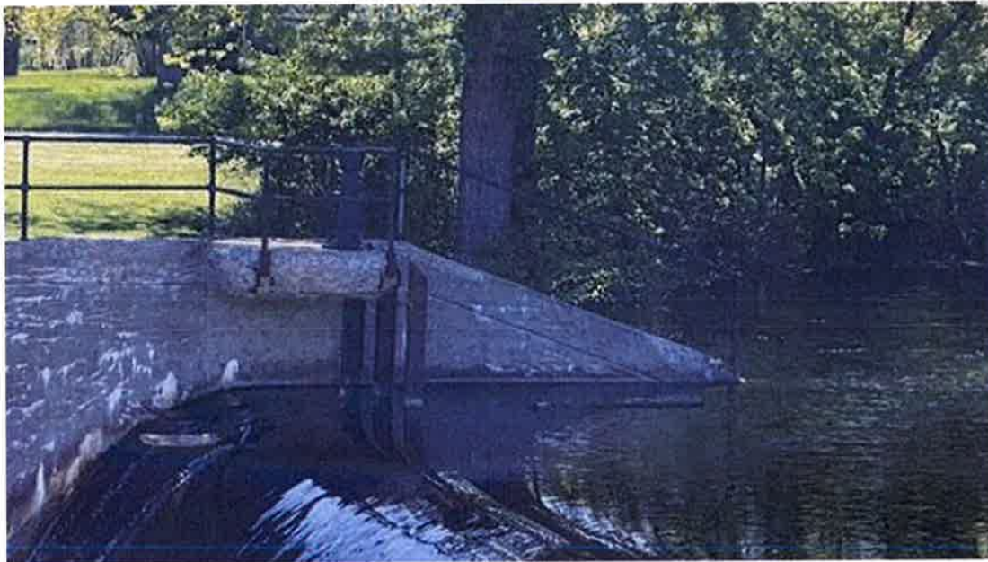
Photo #54 - Right upstream spillway abutment wall. Also note deterioration of gate operator deck
