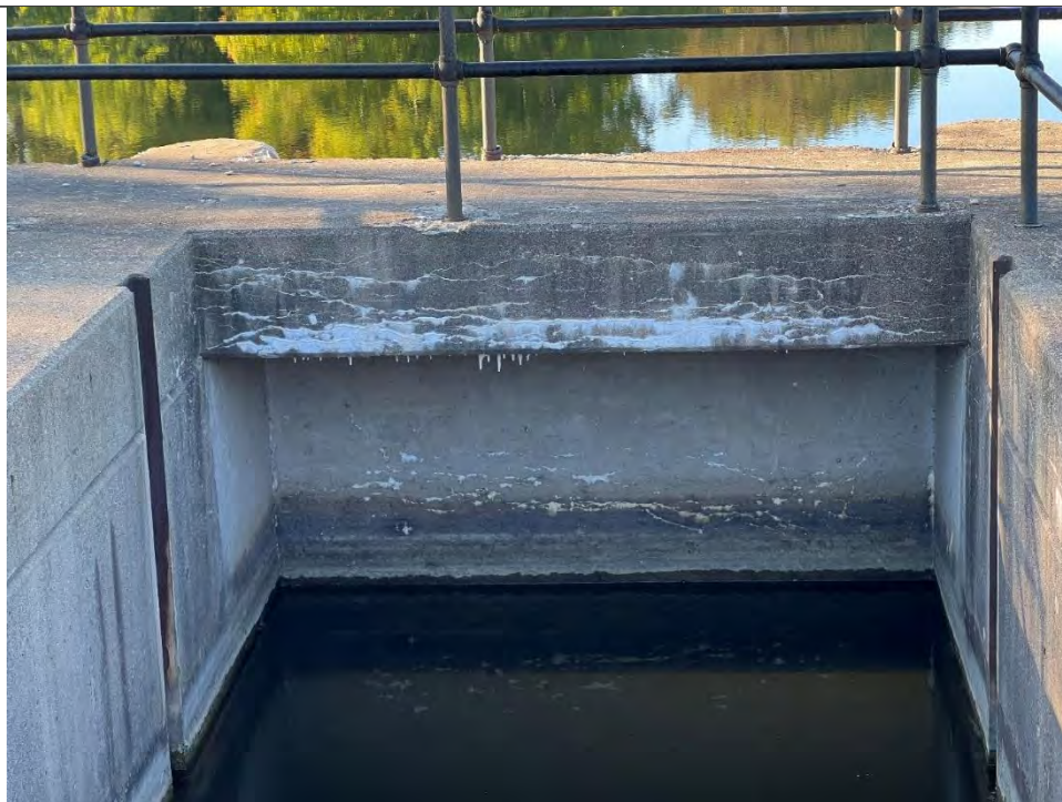
Photo No. 38 – Stoplog Slots in Penstock Intake above Headwater Looking Upstream
