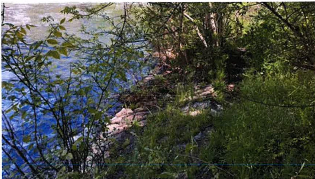
Photo #90 - Right bank of channel downstream of dam across from the powerhouse. Grouted riprap has become overgrown with trees and brush
