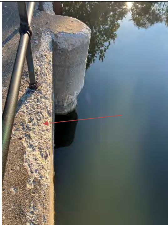
Photo No. 34 – Concrete Deterioration of Upstream Side of Penstock Intake Deck Looking Right
