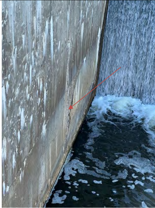
Photo No. 75 – Concrete Deterioration on Face of Downstream Right Wall Upstream of M-52 Bridge Looking Upstream
