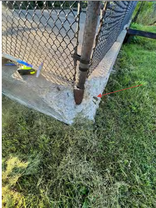
Photo No. 29 – Concrete Deterioration on Downstream Left Corner of Penstock Intake Deck Looking Upstream
