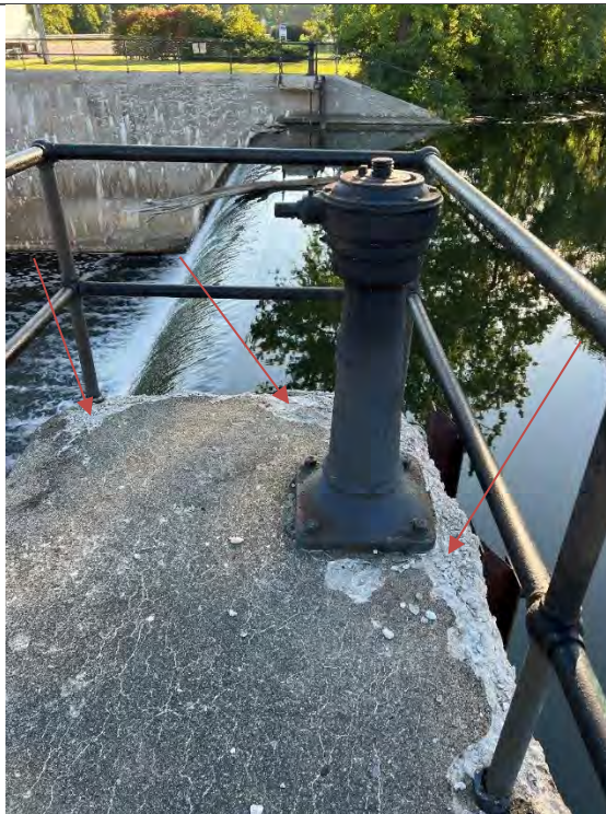
Photo No. 18 – Concrete Deterioration on Right and Upstream Side of Left Operator Deck
