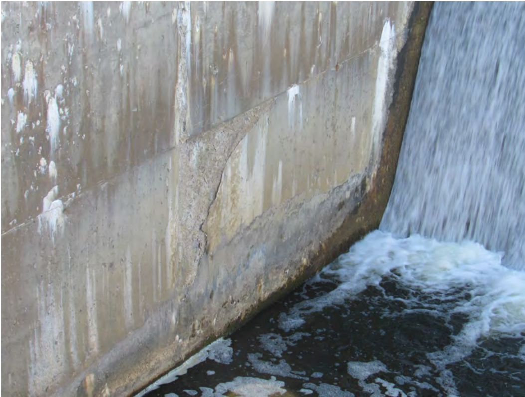
Figure 6 – Downstream, East Wall: Delamination
