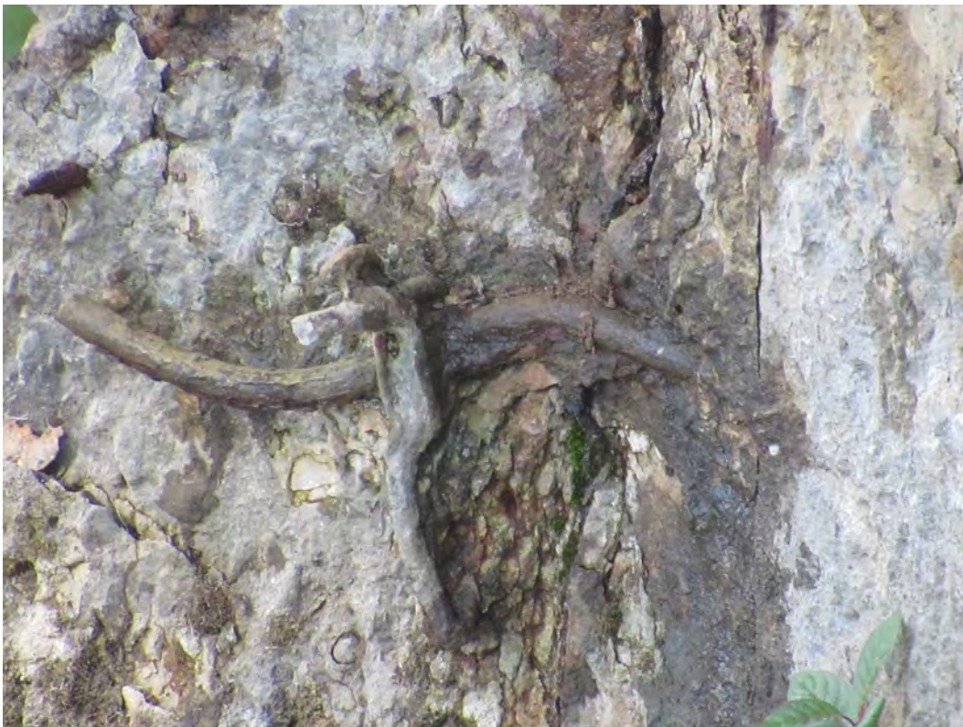
Figure 11 – Downstream, West Wall: Spalling with Exposed Rebar
