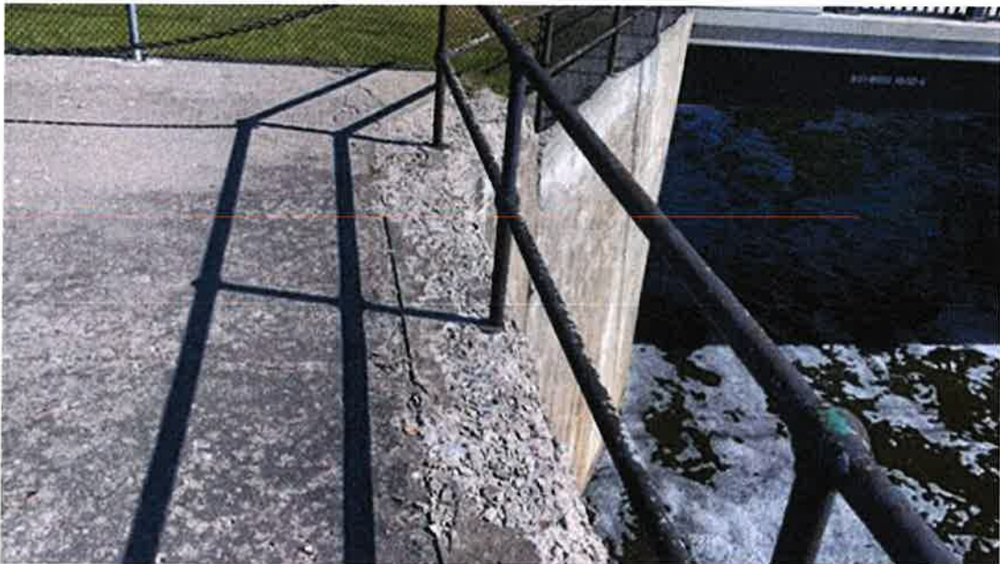
Photo #48 - Spalling on top of left spillway abutment wall
