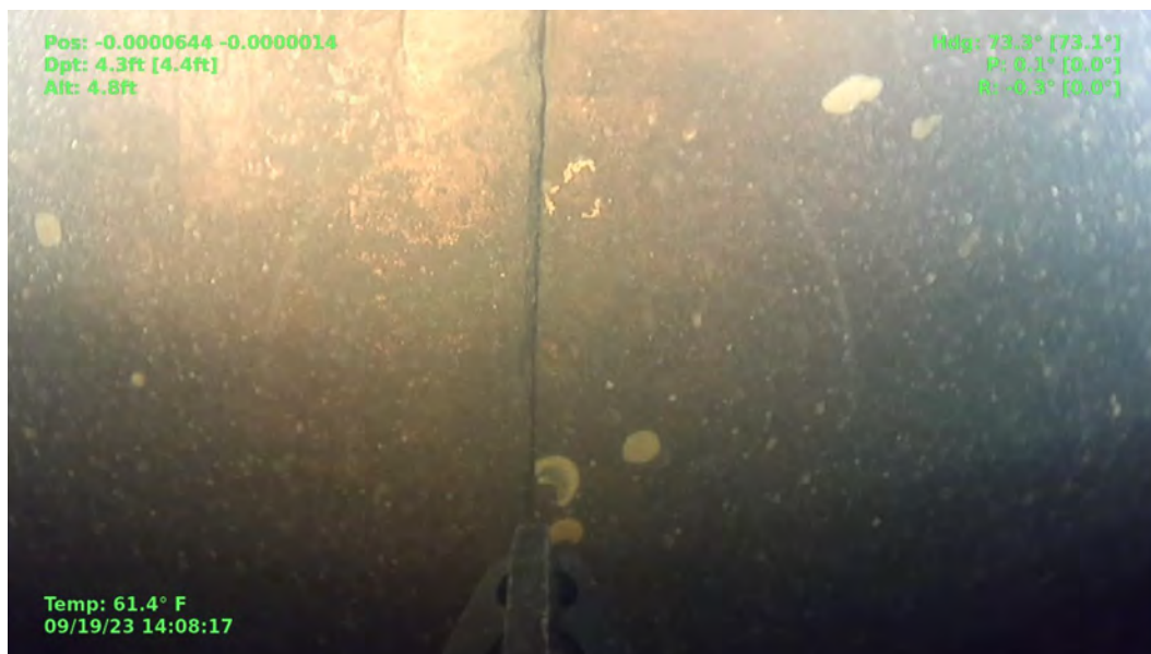
Figure 23 – Upstream, Intake Tunnels East Wall: Construction Joint
