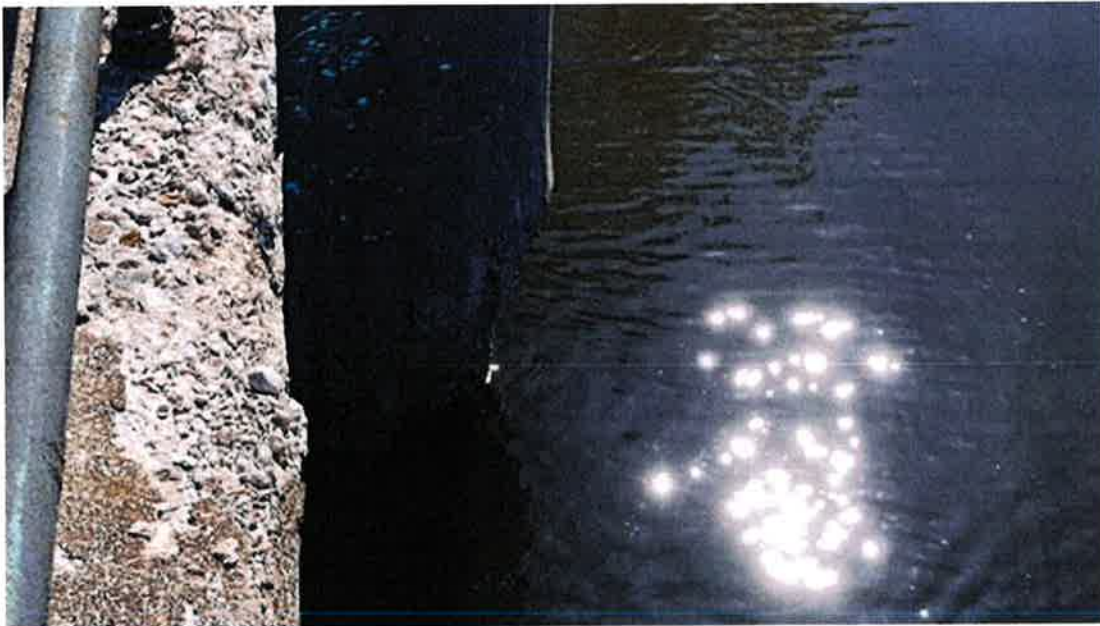
Photo #94 - Loss of concrete at waterline of powerhouse sluiceway inlet, right side
