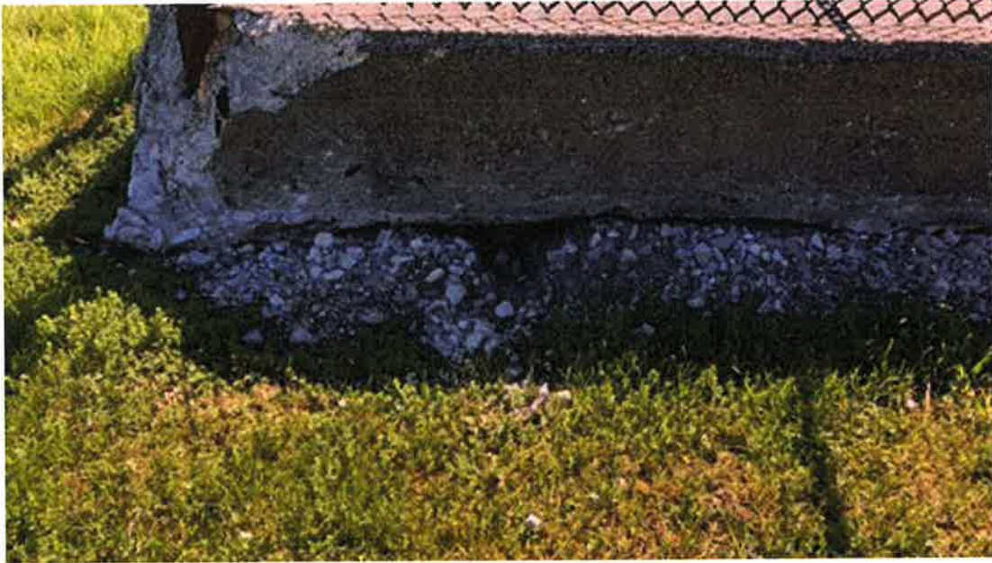
Photo #13 - Burrow observed under spillway concrete at left end of spillway
