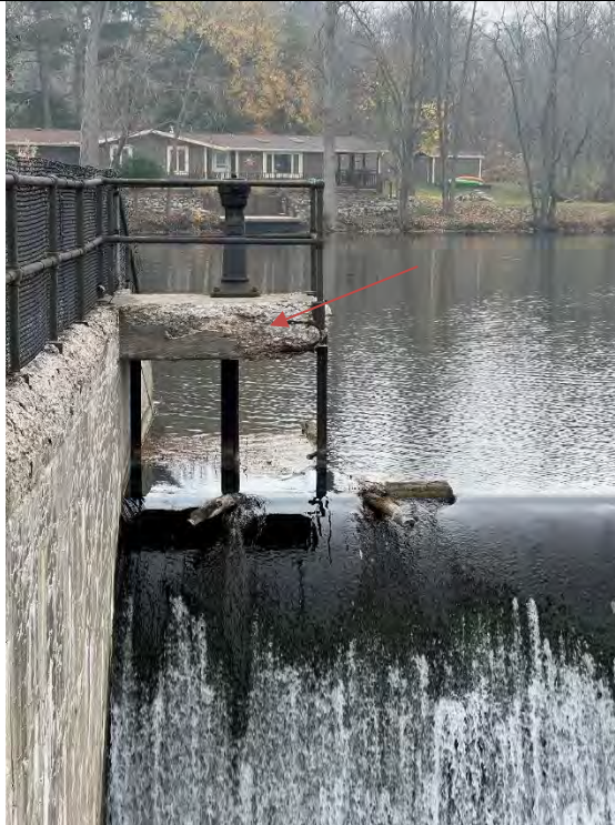
Photo No. 21 – Concrete Deterioration on Downstream Side of Right Operator Deck
