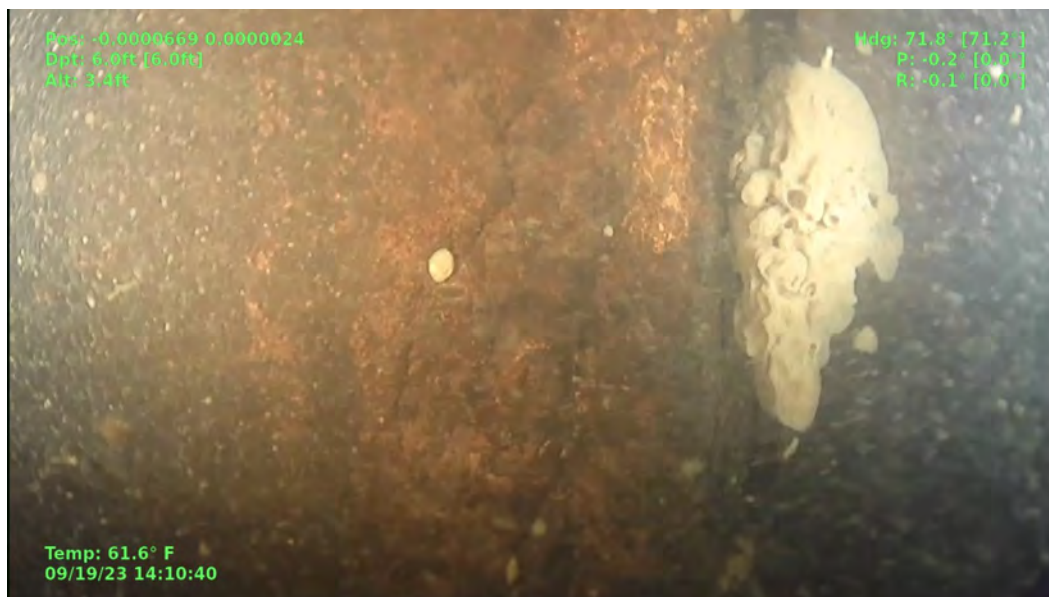
Figure 25 – Upstream, Intake Tunnels East Wall: Spalling on Ceiling
