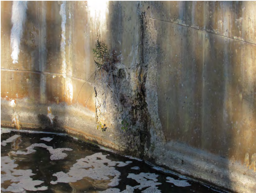
Figure 10 – Downstream, West Wall: Spalling with Exposed Rebar
