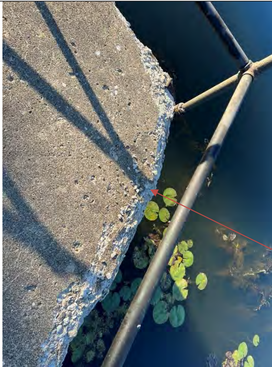
Photo No. 33 – Concrete Deterioration of Upstream Left Corner of Penstock Intake Deck Looking Upstream
