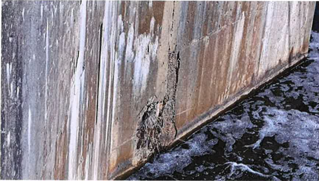
Photo #47 - Cracking and loss of concrete observed near the bottom of the left downstream abutment wall
