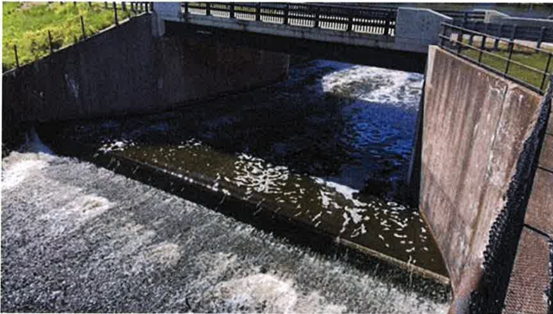
Photo #87 - Spillway outlet and sill
