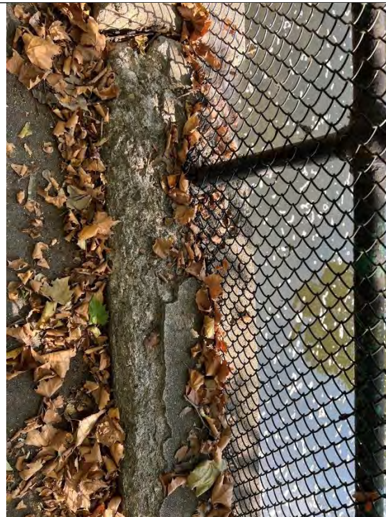
Photo No. 88 – Concrete Deterioration at Top of Seating Area Wall Looking Right
