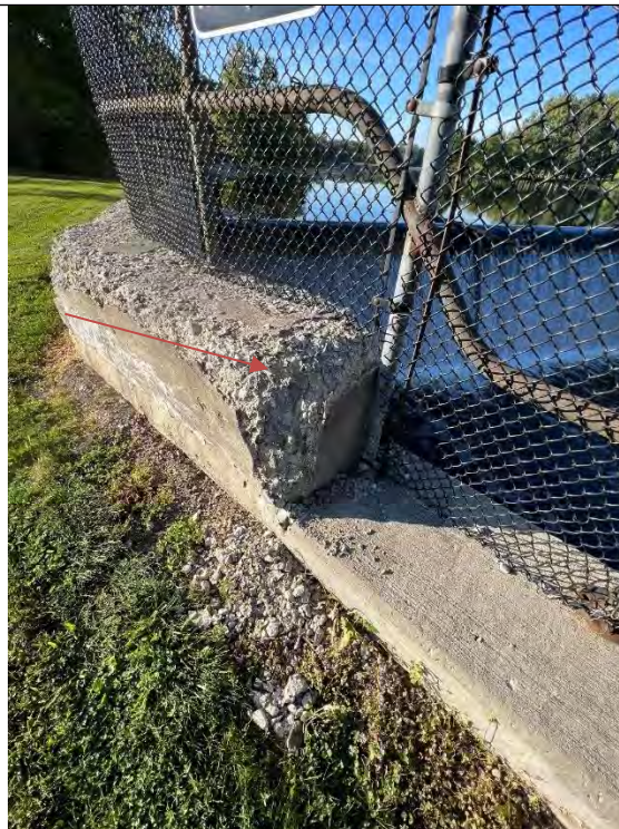
Photo No. 70 – Concrete Deterioration Top of Downstream Right Wall Upstream of M-52 Bridge Looking Upstream
