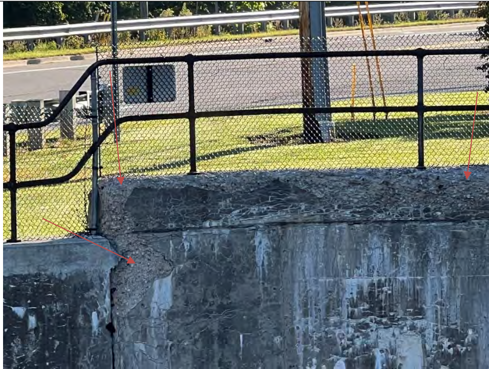
Photo No. 67 – Concrete Deterioration at Top of Downstream Right Wall Upstream of M-52 Bridge Looking Right
