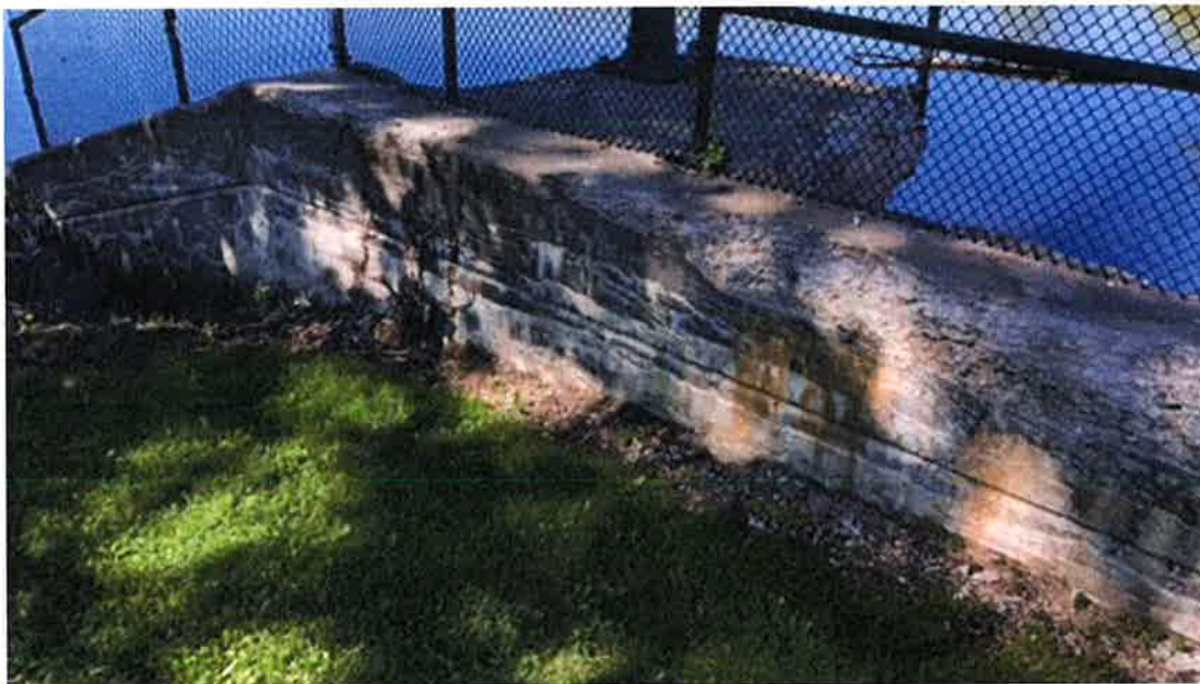
Photo #65 - Spillway right abutment wall right face. Spalling present
