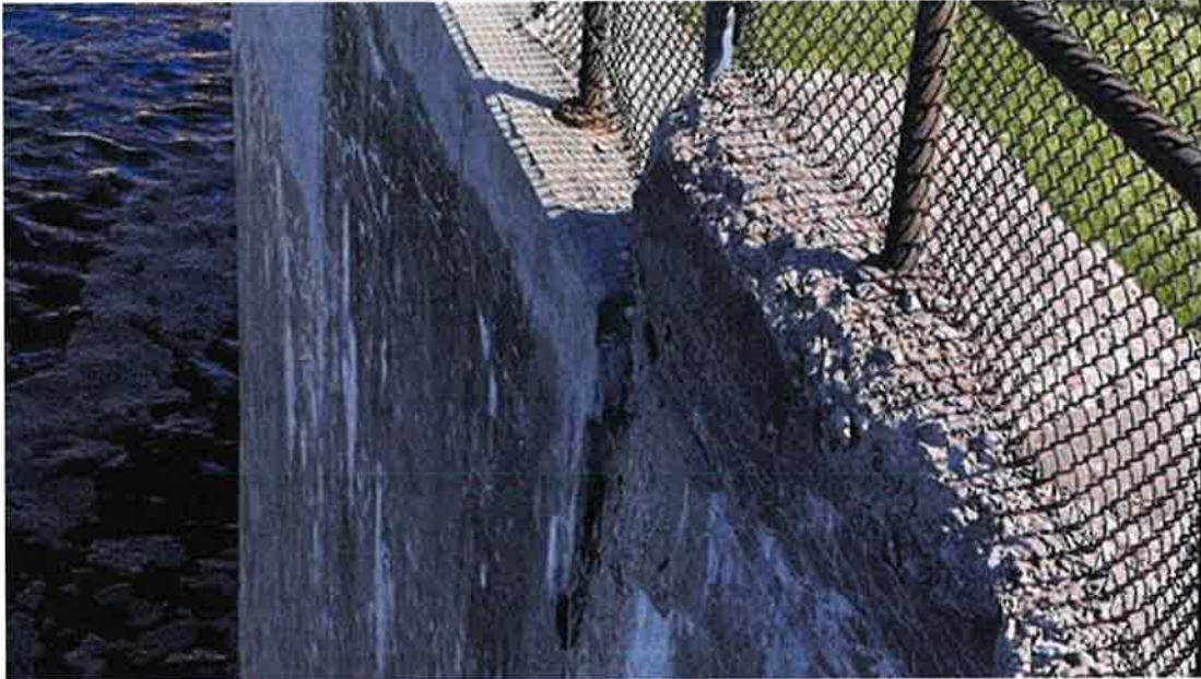
Photo #61 – Concrete deterioration on spillway's right downstream abutment wall
