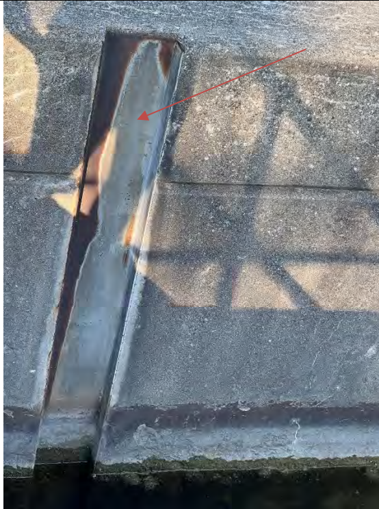
Photo No. 39 – Left Stoplog Slot above Headwater Looking Left
