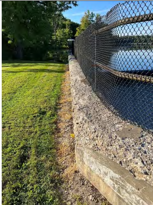
Photo No. 71 – Concrete Deterioration Top of Downstream Right Wall Upstream of M-52 Bridge Looking Upstream
