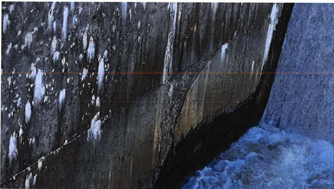
Photo #56 - Concrete delamination on spillway's right downstream abutment wall
