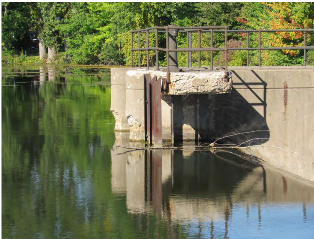
Figure 18 – Upstream, West Sluice Gate and Intake Tunnel
