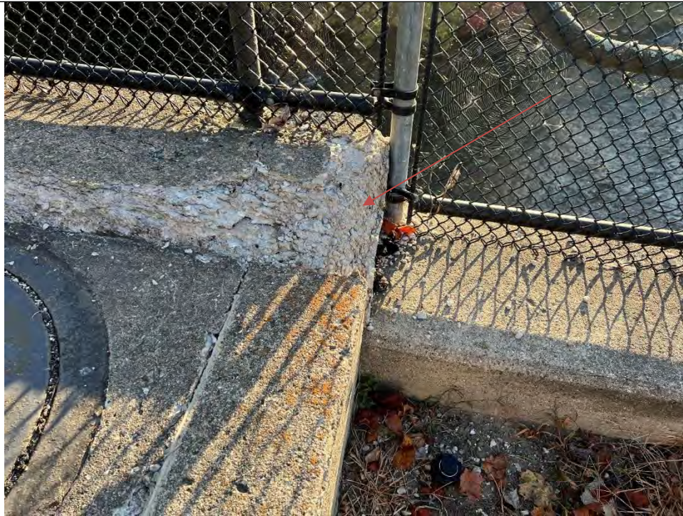
Photo No. 53 – Concrete Deterioration at Top of Downstream Left wall Upstream of Powerhouse Looking Right
