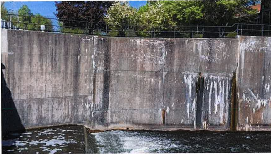
Photo #77 - Spillway left downstream abutment wall downstream of bridge. Some efflorescence present. Seepage observed
