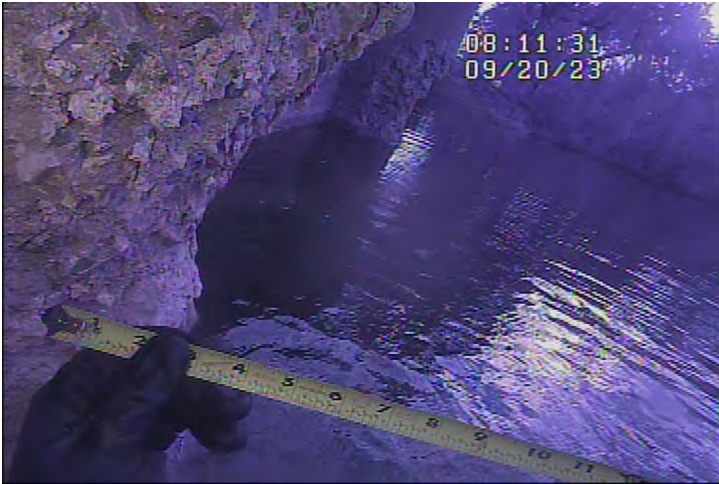
Figure 36 – Upstream, Intake Tunnel Bullnose 2: Concrete Loss
