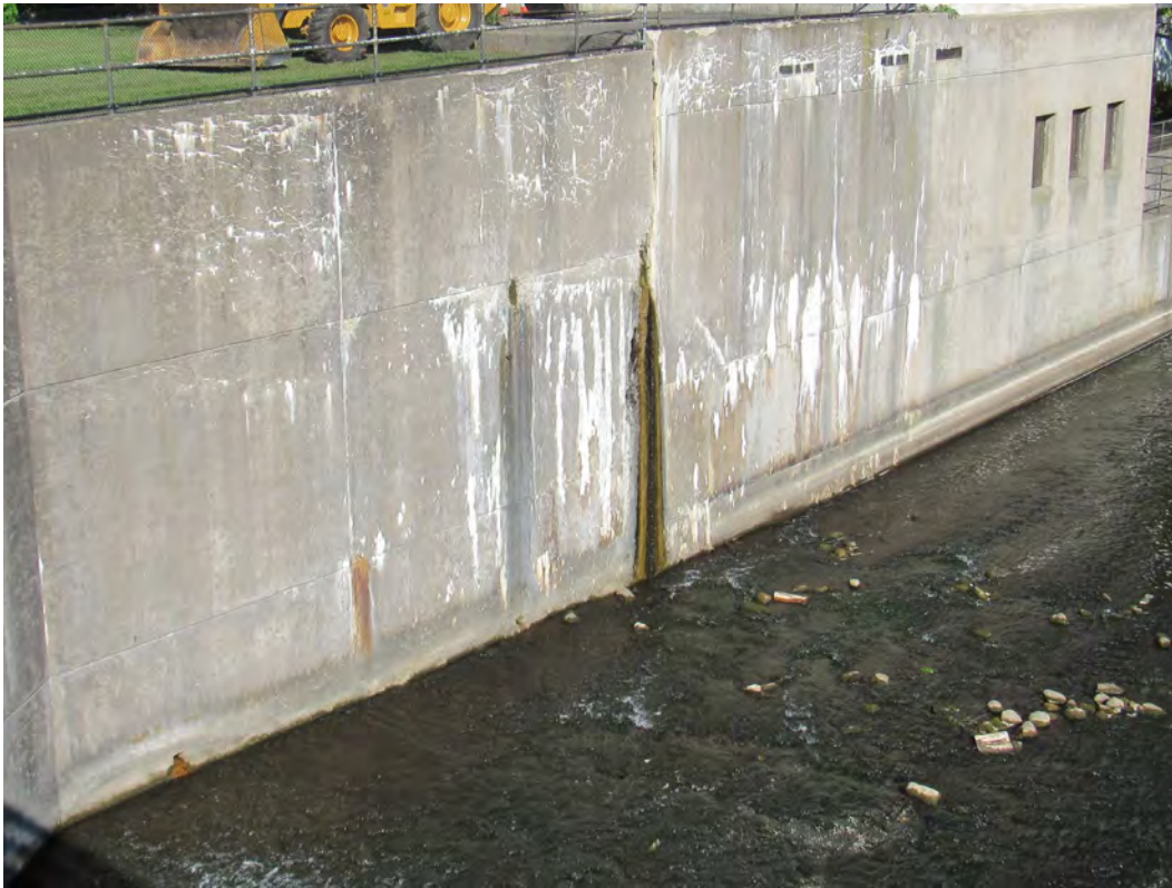
Figure 12 – Downstream, West Wall: Spalled Out Construction Joint
