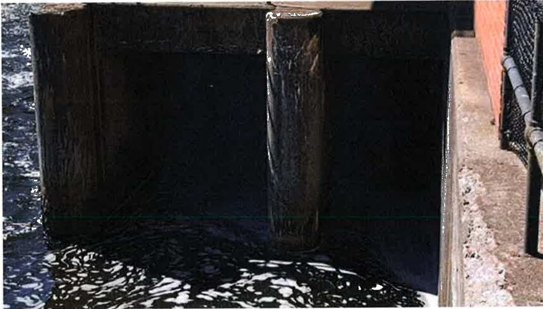
Photo #97 - Powerhouse outlet. Efflorescence present on concrete piers
