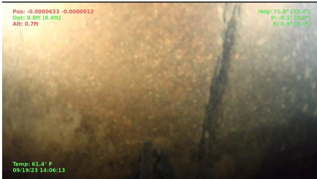
Figure 22 – Upstream, Intake Tunnels East Wall: Construction Joint
