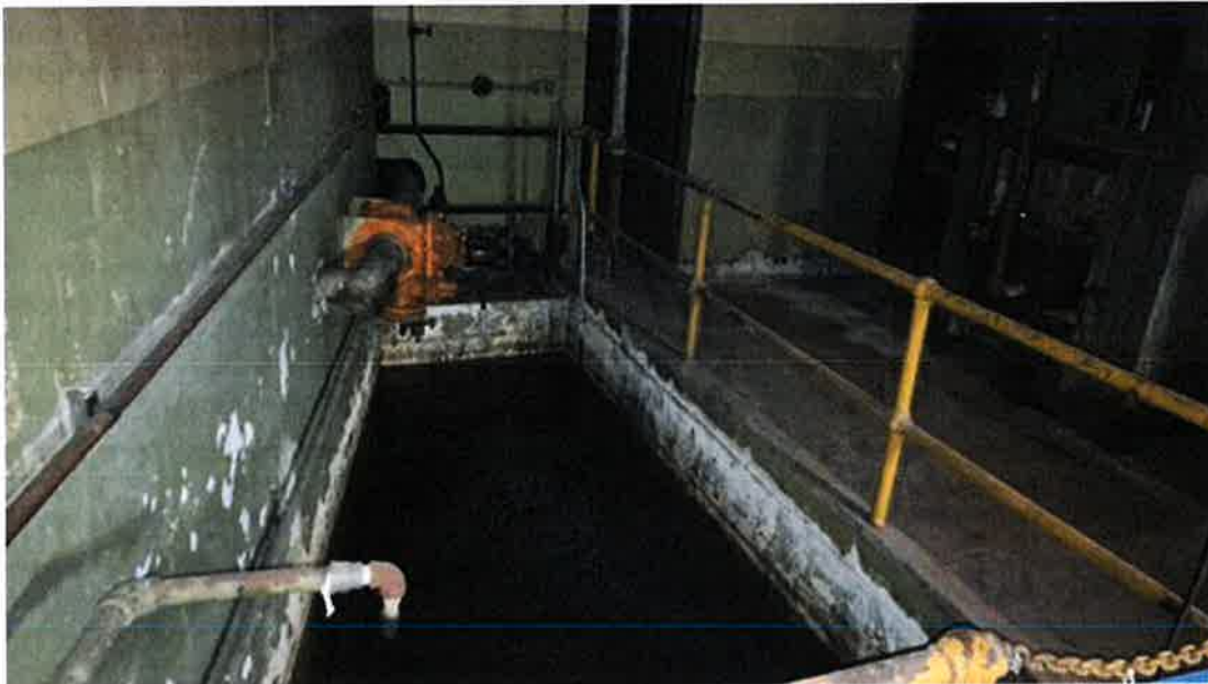
Photo #102 - Sluiceway in basement of powerhouse
