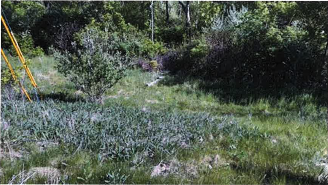
Photo #27 - Downstream slope of right embankment viewed from crest. Some brush is present and encroaching upward beyond toe
