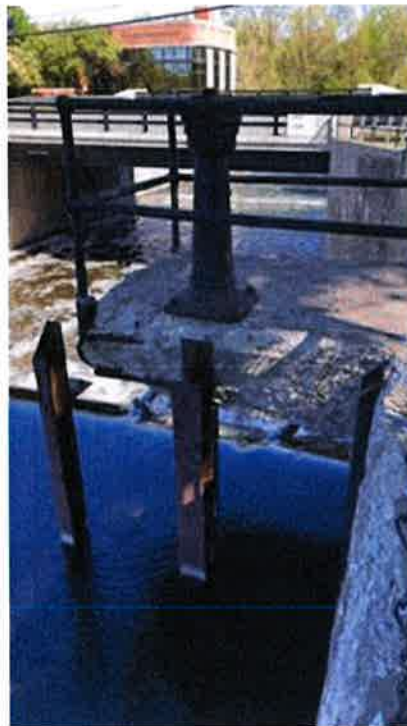
Photo #70 - Right drawdown gate operator. Note severe deterioration of concrete on operator deck
