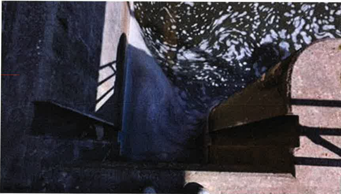
Photo #96 - Previous powerhouse outlet into river. No water currently flows through sluiceway
