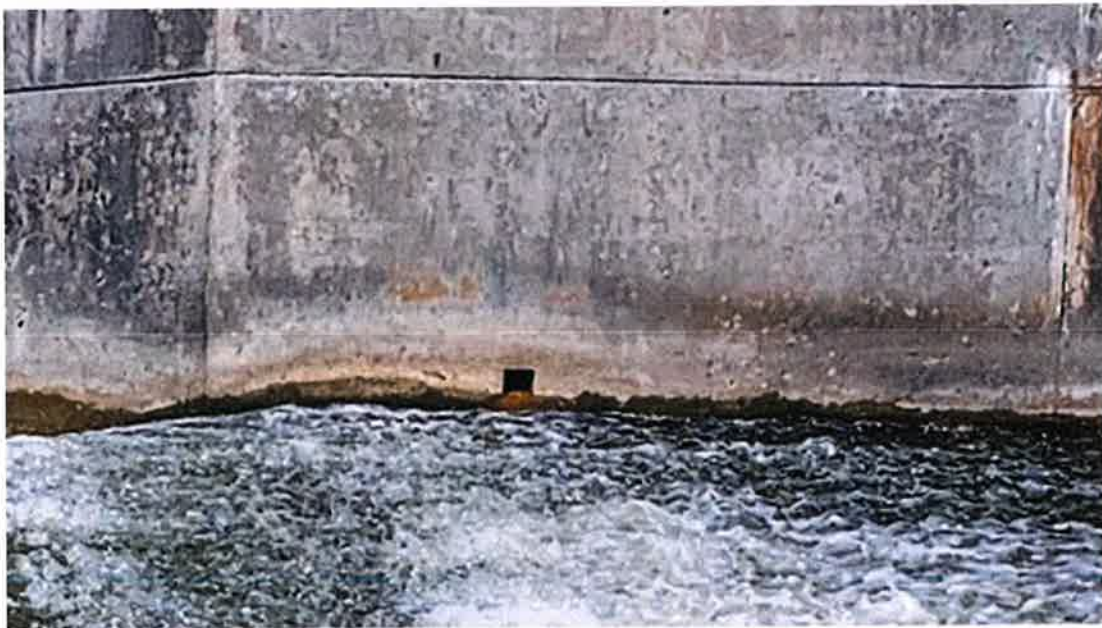
Photo #78 - Wall drain on left downstream abutment wall
