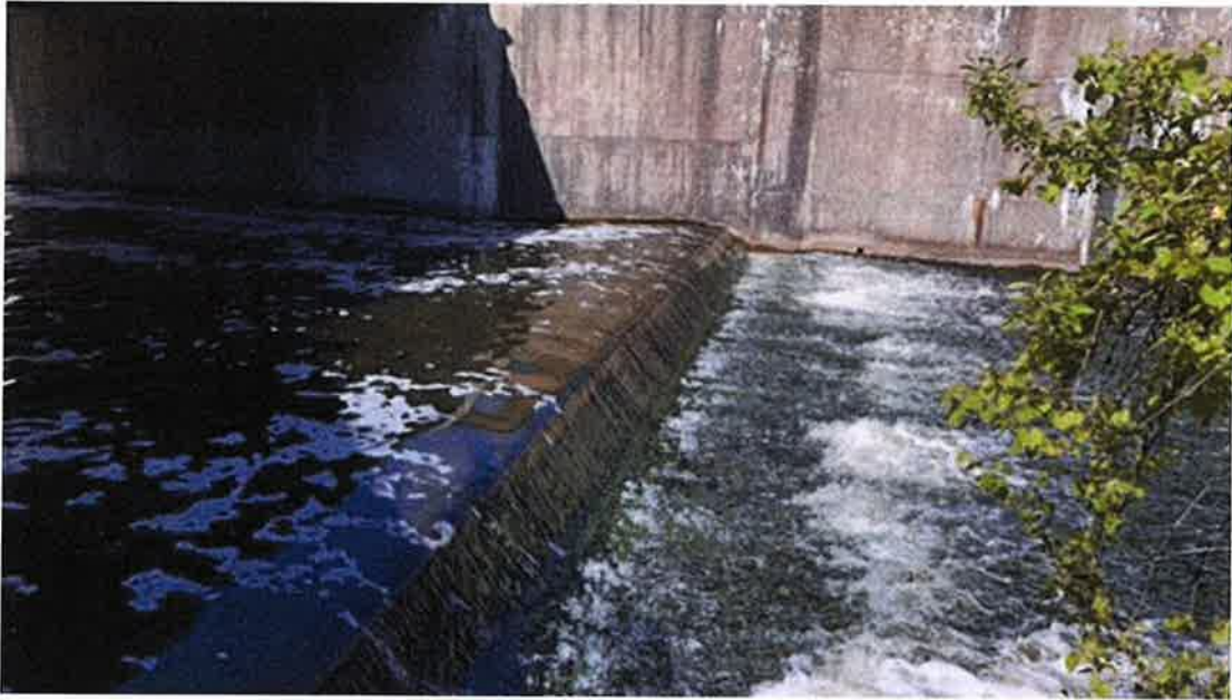
Photo #75 - Spillway sill downstream of bridge
