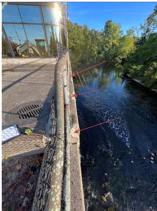
Photo No. 62 – Concrete Deterioration on Top of Downstream Left Wall Downstream of M-52 Bridge Looking Downstream
