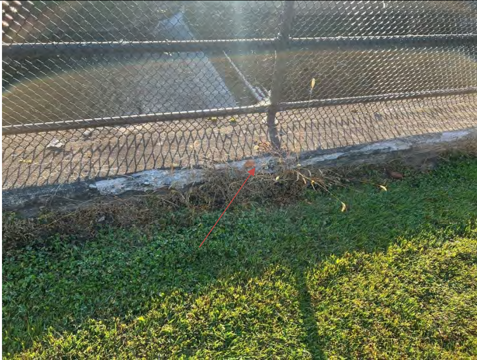
Photo No. 55 – Concrete Deterioration at Top of Downstream Left Wall Downstream of M-52 Bridge Looking Right
