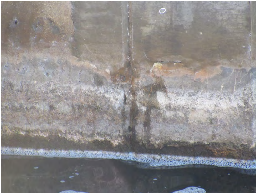
Figure 5 – Downstream, East Wall: Spalling
