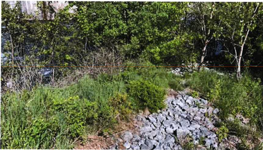
Photo #32 - Storm sewer outfall downstream flow path. Some of the flow path has been armored. Downstream of the armoring in the photo, runoff gullies are present
