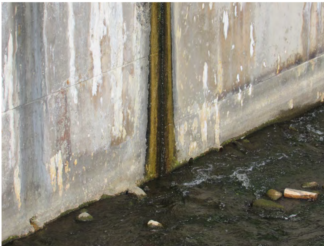
Figure 14 – Downstream, West Wall: Spalled Out Construction Joint
