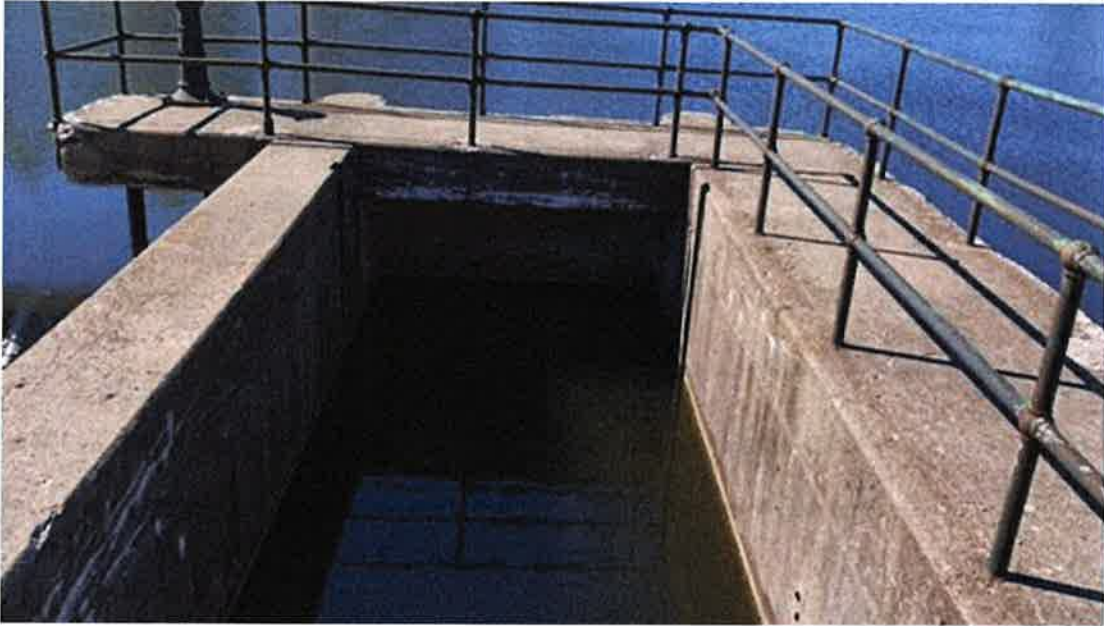
Photo #99 - Sluiceway inlet adjacent to principal spillway, looking upstream
