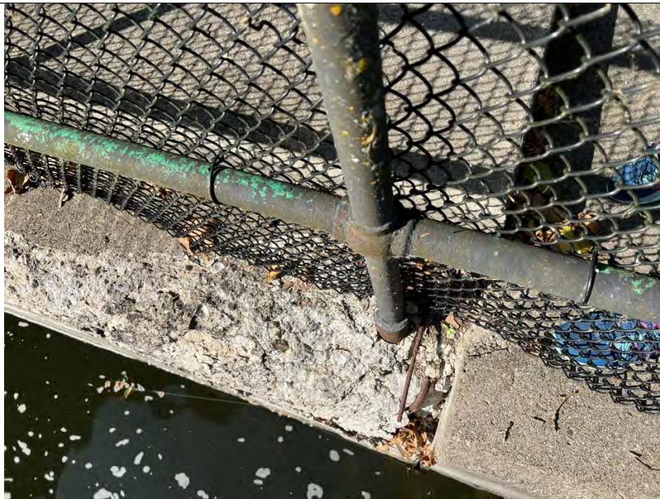
Photo No. 86 – Concrete Deterioration at Top of Seating Area Wall Looking Left
