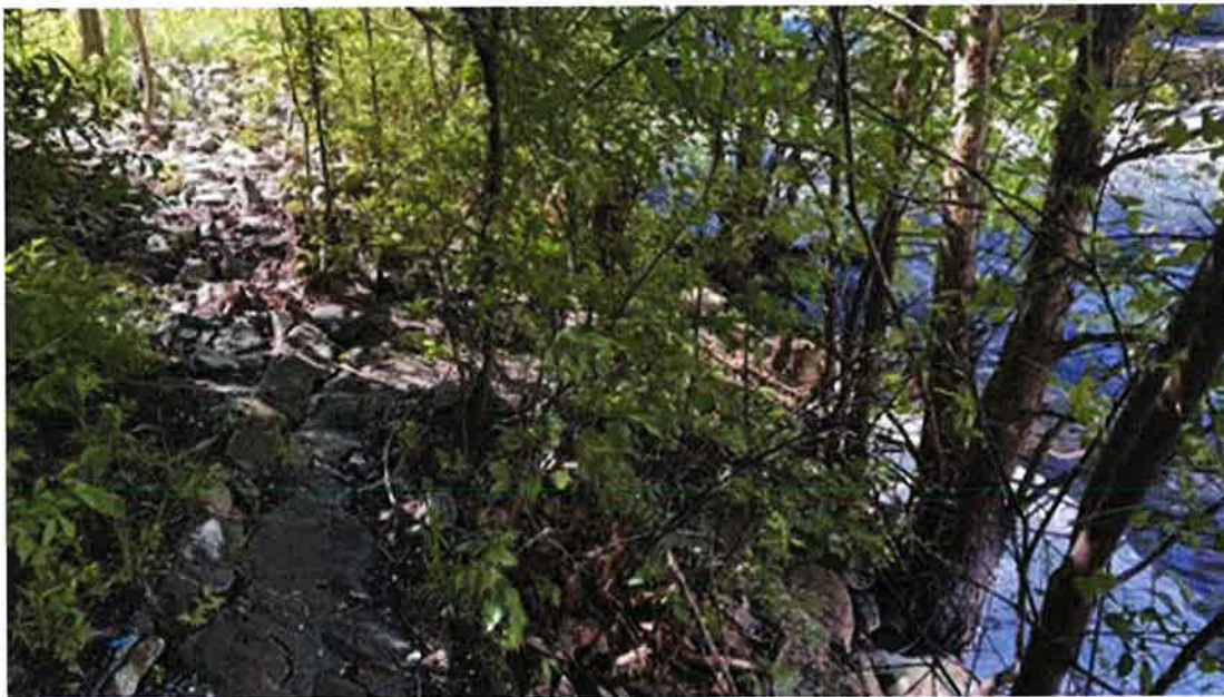
Photo #89 - Right bank of channel downstream of dam across from the powerhouse. Grouted riprap has become overgrown with trees and brush
