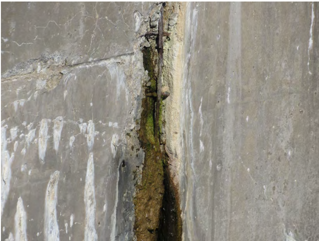
Figure 13 – Downstream, West Wall: Spalled Out Construction Joint: Exposed Rebar
