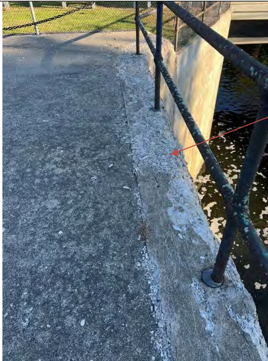
Photo No. 35 – Concrete Deterioration of Right Side of Penstock Intake Deck Looking Downstream
