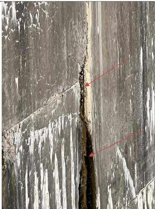
Photo No. 50 – Concrete Deterioration and Leaking at Construction Joint on Downstream Left Wall Downstream of M-52 Bridge
